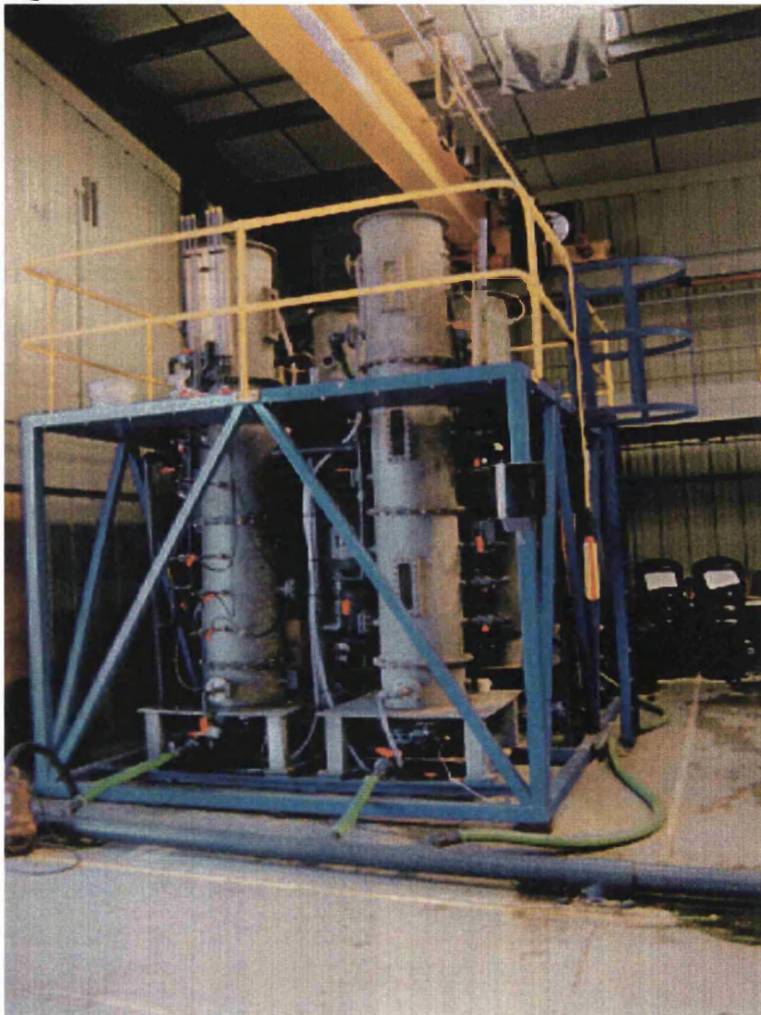
Figure 5.7: Pilot Columns at Manor Farm STW
