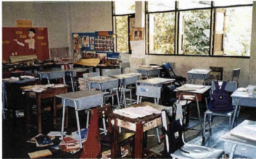
Figure A12.5 Conditions of windows and classroom; fair windows (no safety catches or frame but the lower border of windows is high above floor [at least 1 metre]) and poor cleanliness of classroom (rubbish and untidy)
