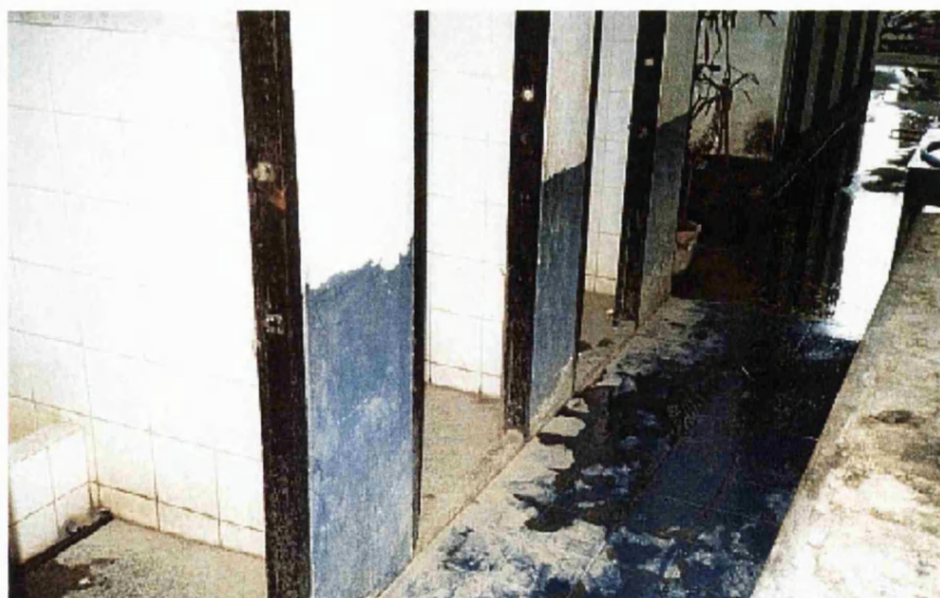
Figure A12.16 Conditions of toilets; poor cleanliness of toilets (sand and wet) and poor floor surface of toilets (slippery and with risky steps)
