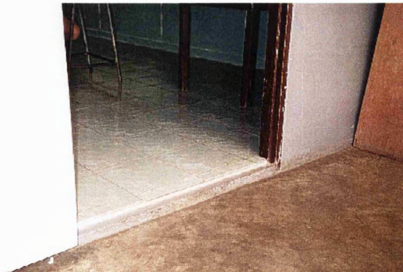
Figure A12.8 Condition of classroom; poor floor surface of classroom (slippery and with risky step)
