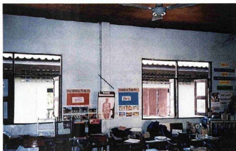
Figure A12.2 Condition of windows; fair windows (no safety catches or frame, but the lower border of windows is high above floor [at least 1 metre])
