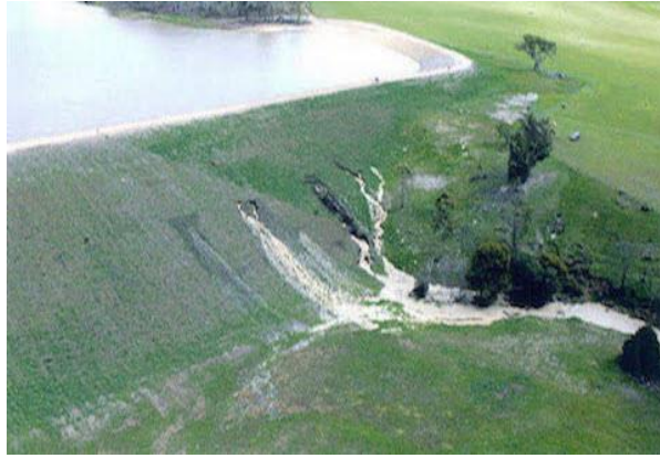
Figure 98 A dam failure by piping in Tunbridge dam, Tasmania, Australia (source: Wrachien and Mambretti, 2009)
