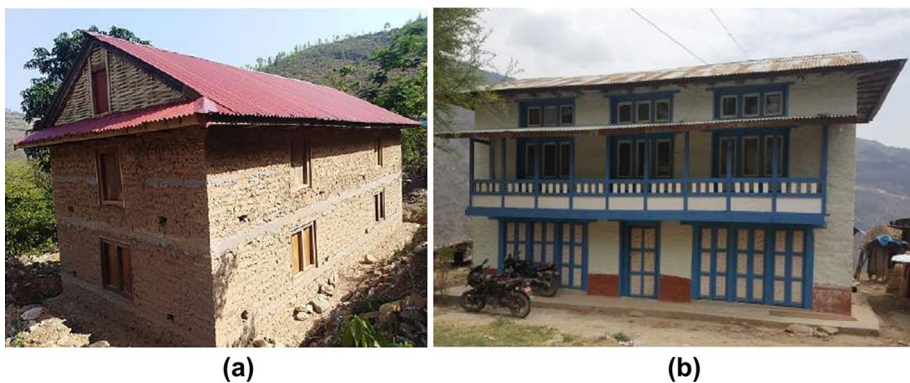
Fig. 5 Photographs of multi-storeyed non-compliant SMM houses built with limited (or without) NRA technical assistance: a photo from Sindhuli and b photo from Solukhumbu (HRRP 2018). In these houses, the seismic bands are not placed at the recommended spacings (Images reproduced with kind permission of HRRP Nepal)
