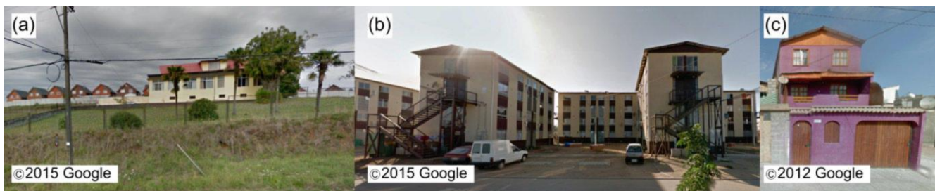
Fig. 7 – The identification of features of different structures during the remote surveys was hampered by the lack of better digital images or the presence of coating (Source: (a) https://goo.gl/maps/noJw6FYGkxA2 ; (b) https://goo.gl/maps/rFSHWTS2PaP2 ; (c) https://goo.gl/maps/R2JCEejQUkr )
