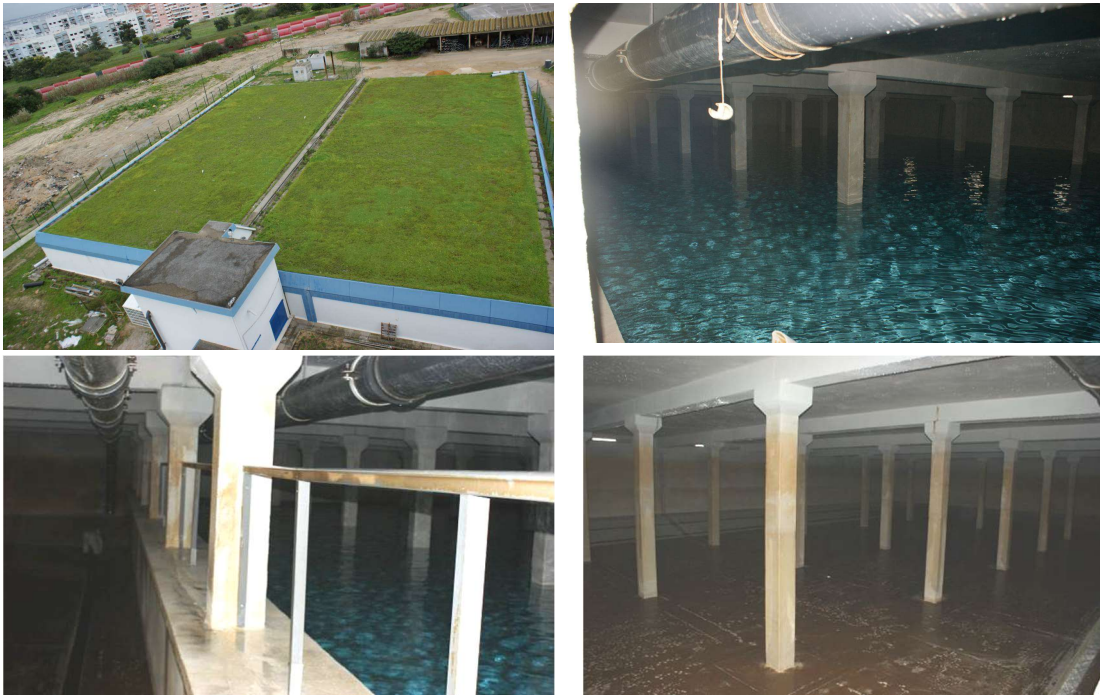
Figure 1. Photographs from the interior and exterior of the studied water tank.
