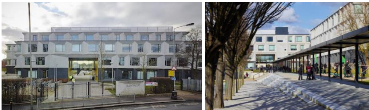
Figure 1: Case study school; (Left) Entrance – West façade, (Right) Central courtyard.
