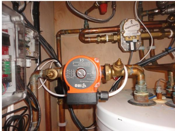
**Fig. 1.** CS12 – Uninsulated pipework associated with heat pump.
