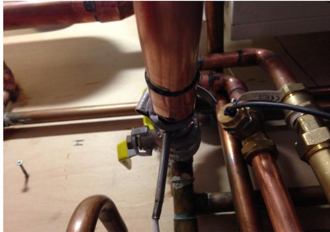
**Fig. 2.** CS12 - pipework showing insulation between temperature sensor and pipe. The auxiliary temperature sensor for the heat meter is just right-of-centre in a pocket. Source, BRE.
