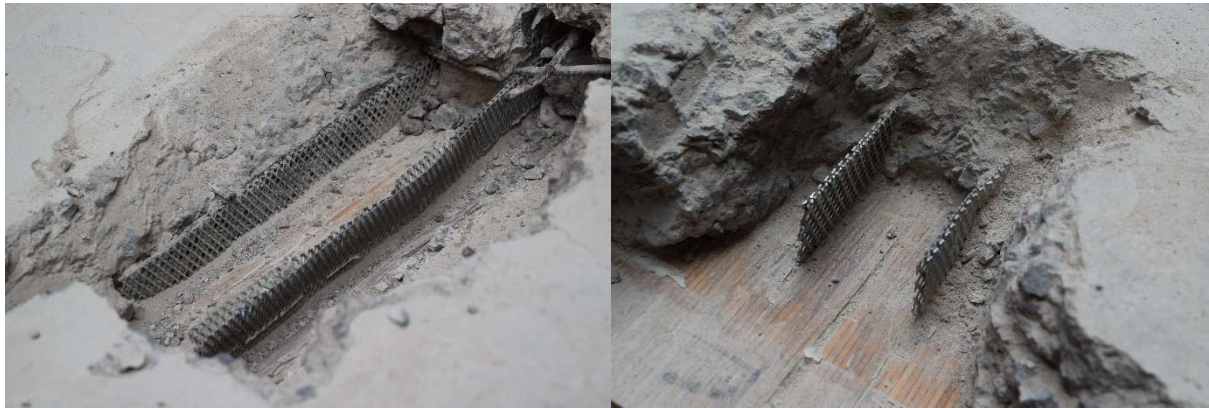
Figure 22 - Post-test observation of (a) central connector on joist J2, and (b) end connector on joist J2.
