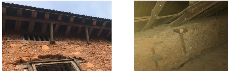
Figure 5. Timber roofing system with timber keys and compression struts: outside view (left) and inside view (right).
