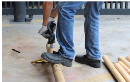
Figure 5: Cutting of culm ends.
