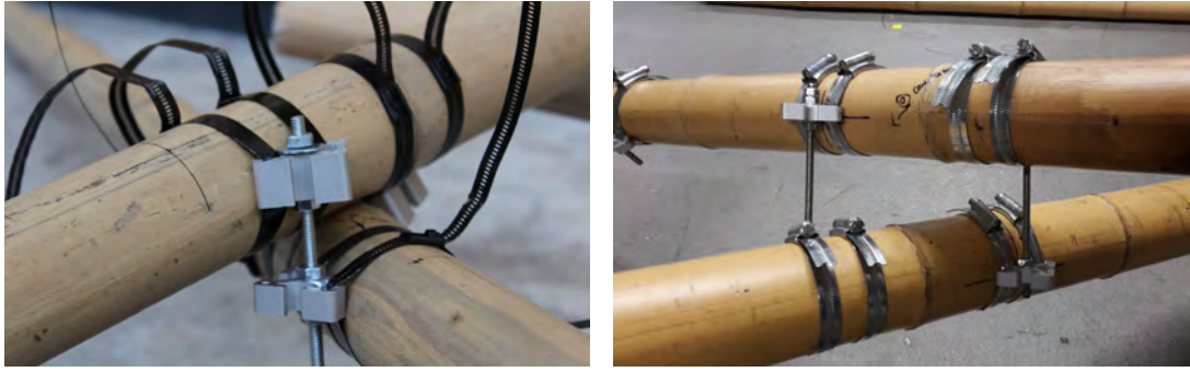
Figure 25: Assembly of aluminium connection with banding system and worm drive steel hose clips.
