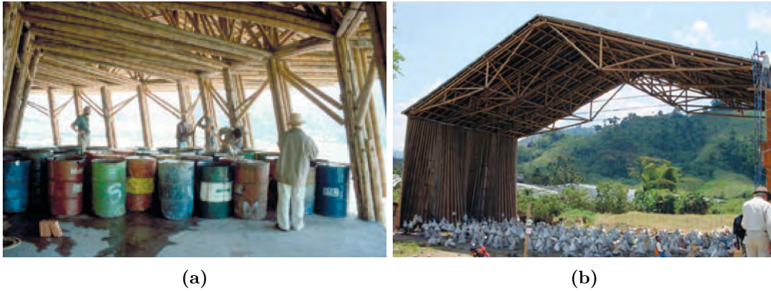
Figure 1.4: Experimental tests. (a) Full scale ZERI pavilion in Colombia, and (b) full scale section prototype of the nomadic museum pavilion (Minke, 2012).
