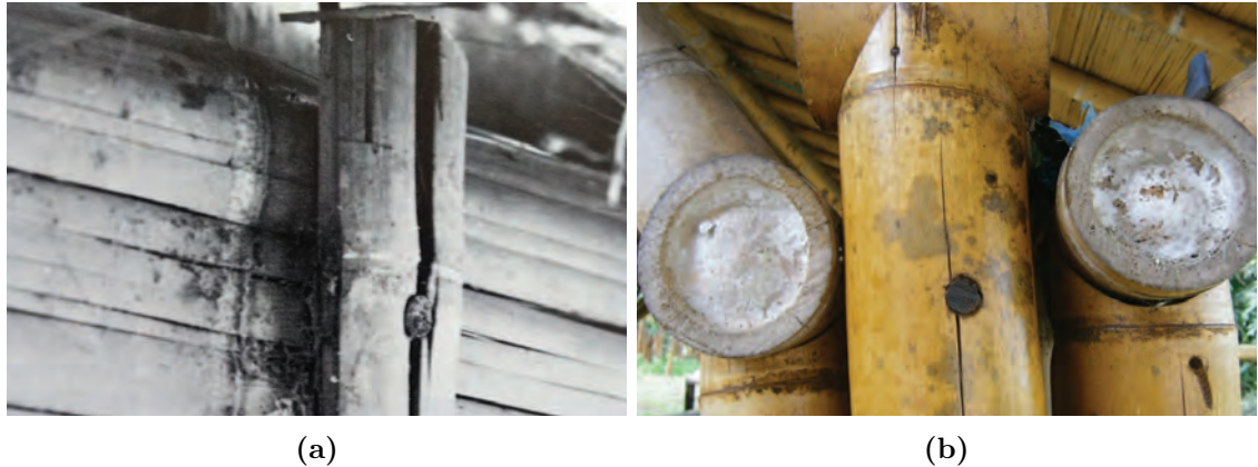
Figure 1.6: (a) Splitting of bamboo culm in connection (Dunkelberg, 1985). (b) Cracked culm in location of dowel rod.
