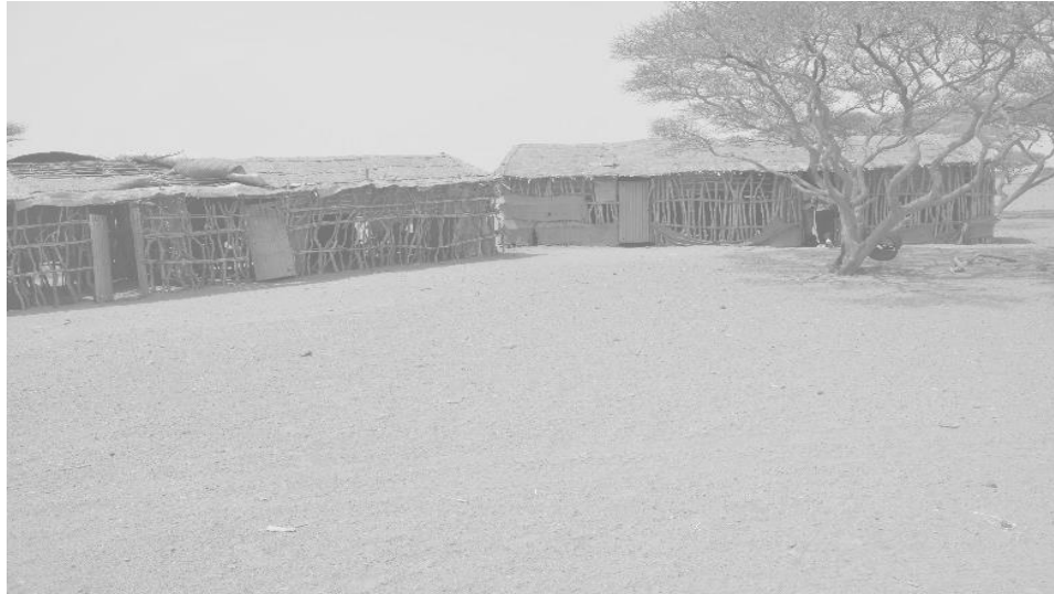
Figure 14 Additional learning spaces constructed by the community at Beles School
