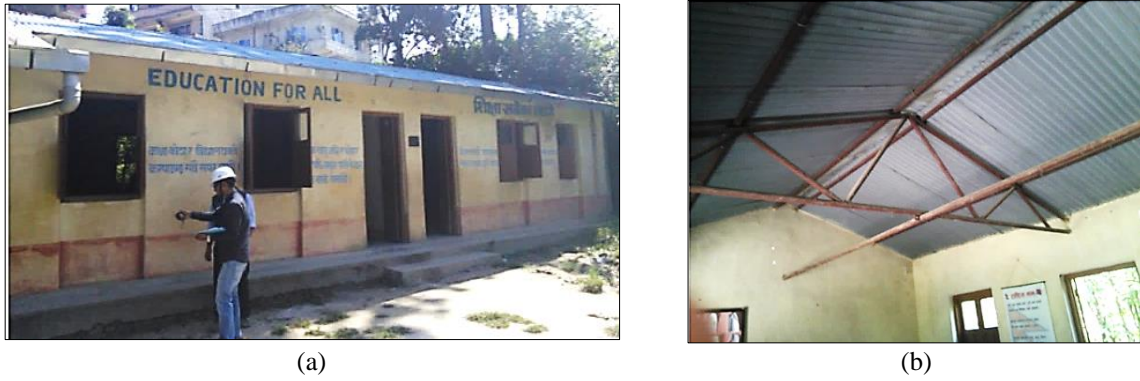
Figure 4: Photographs representative of the case study URM school building: (a) outside front view and (b) Inside view showing the short walls with gables and light steel roof structure. (Image Copyright: The World Bank)
