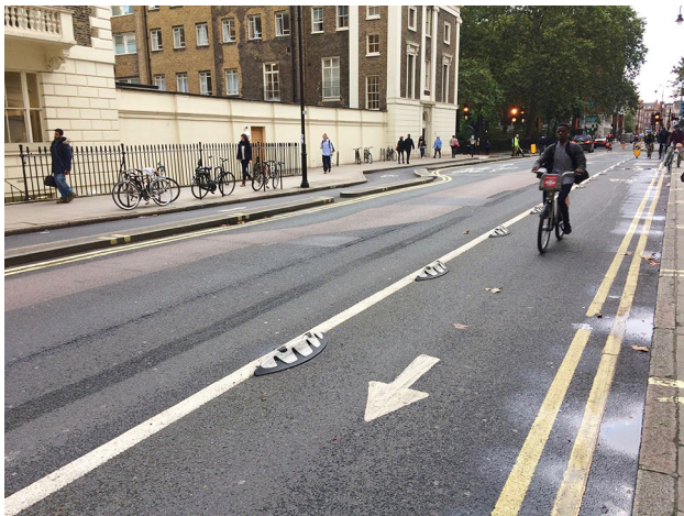
Fig. 7 Exploratory cycleway layouts (to the right of the image) in London's Bloomsbury, implemented at minimal cost prior to more permanent investments (to the left of the image) being made (Matthew Carmona)
