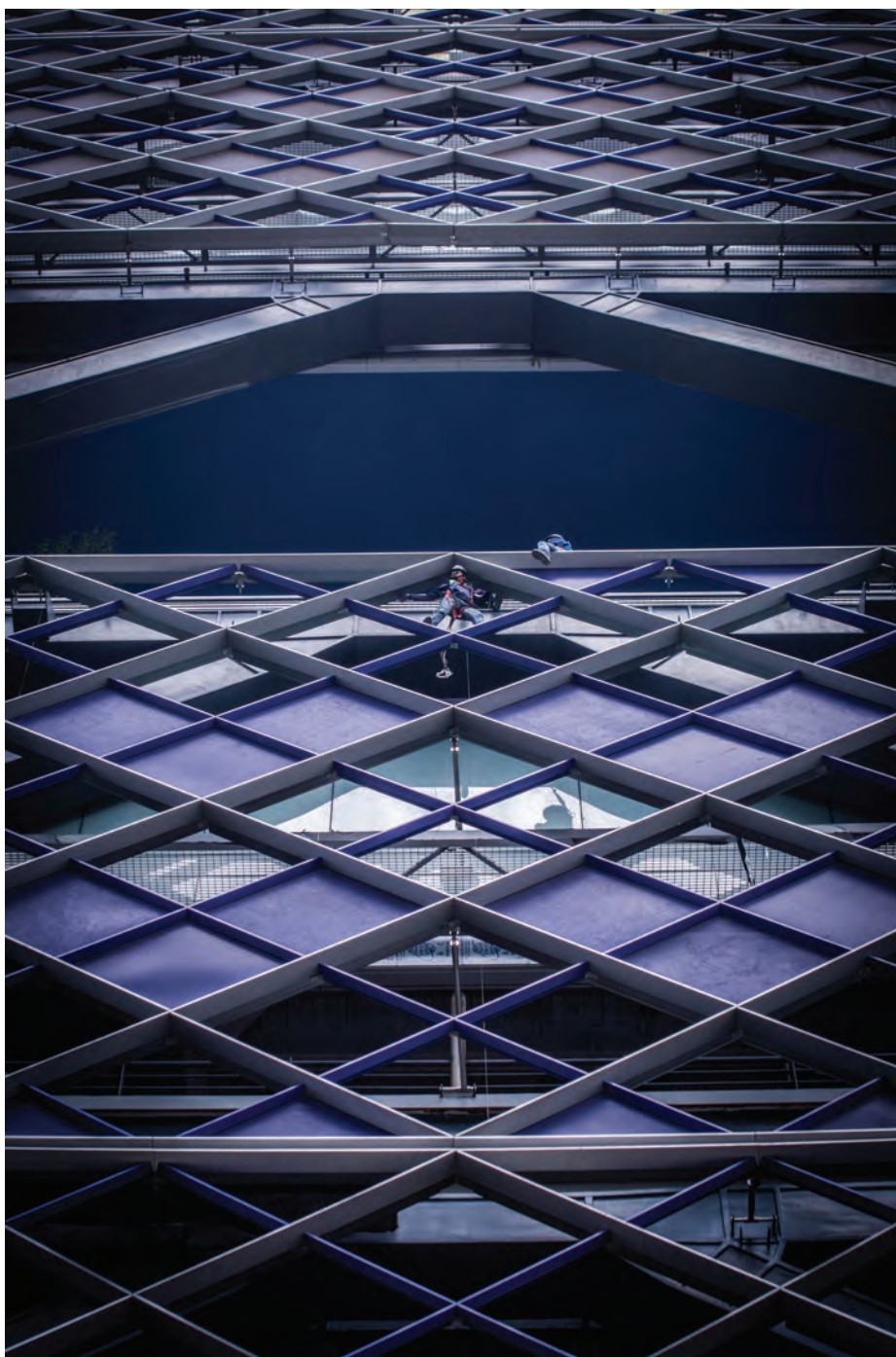
Figure 4. The "Fuse." Expression of this key element could be accomplished by thoughtful arrangement of stiffeners of the oncoming bracing diagonals and beam horizontals. (Source: Rogers Stirk Harbour+Partners)
