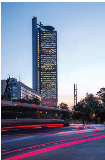
Figure 1. The External steelwork system – the so called Megaframe – is clearly legible form outside, as are the garden spaces formed by the structure. (Source: Mark Gorton, Rogers Stirk Harbour+Partners) 图1. 外部钢架系统，即巨型框架结构，外部形态清晰可辨，这种结构也形成了花园空间。 (来源: Mark Gorton, Rogers Stirk Harbour+Partners)
