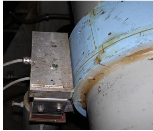
(b) Power meter
