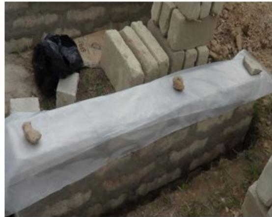
Fig 2 (a) Schematic diagram of the position of the dpc (b) Photograph showing how the dpc was laid (Source: Agyekum et al., 2016)
