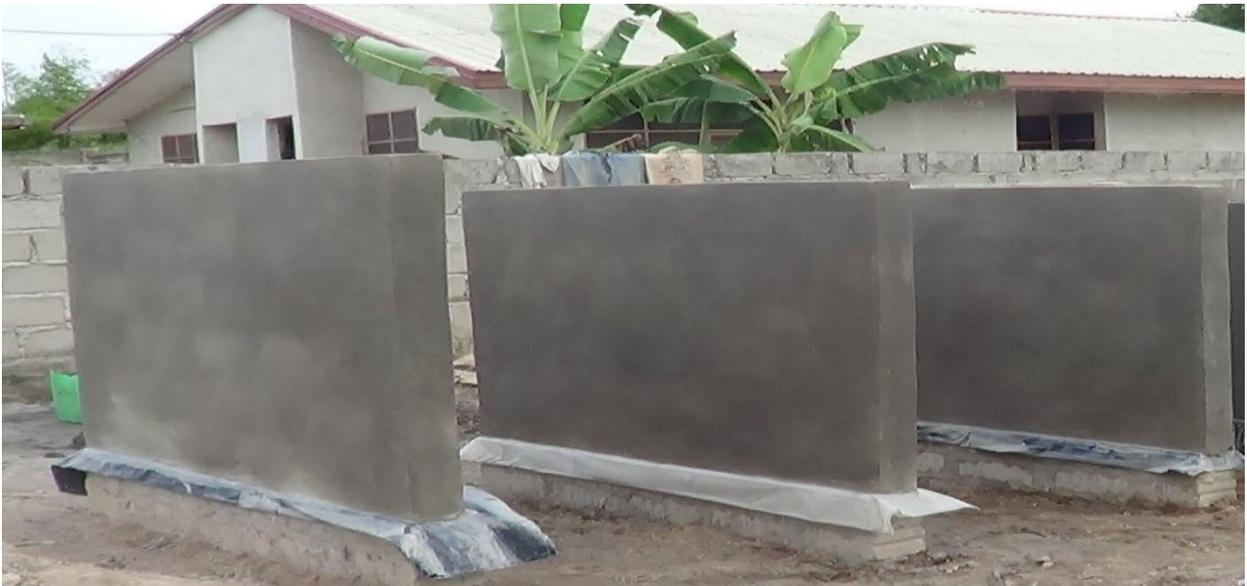
Fig 3 Photograph of test walls after the dpcs were laid
