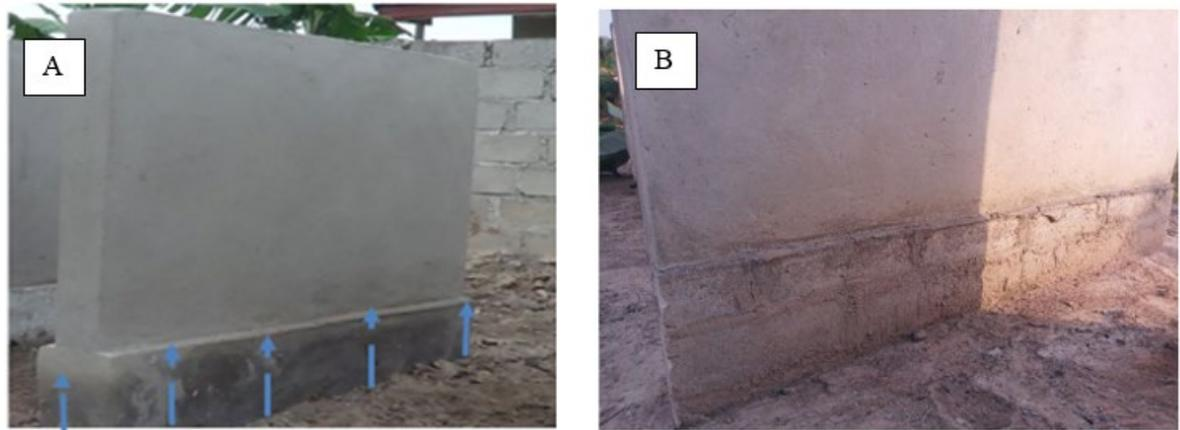
Fig 15 Photographs showing the presence (left) and absence (right) of water at the bases of the walls
