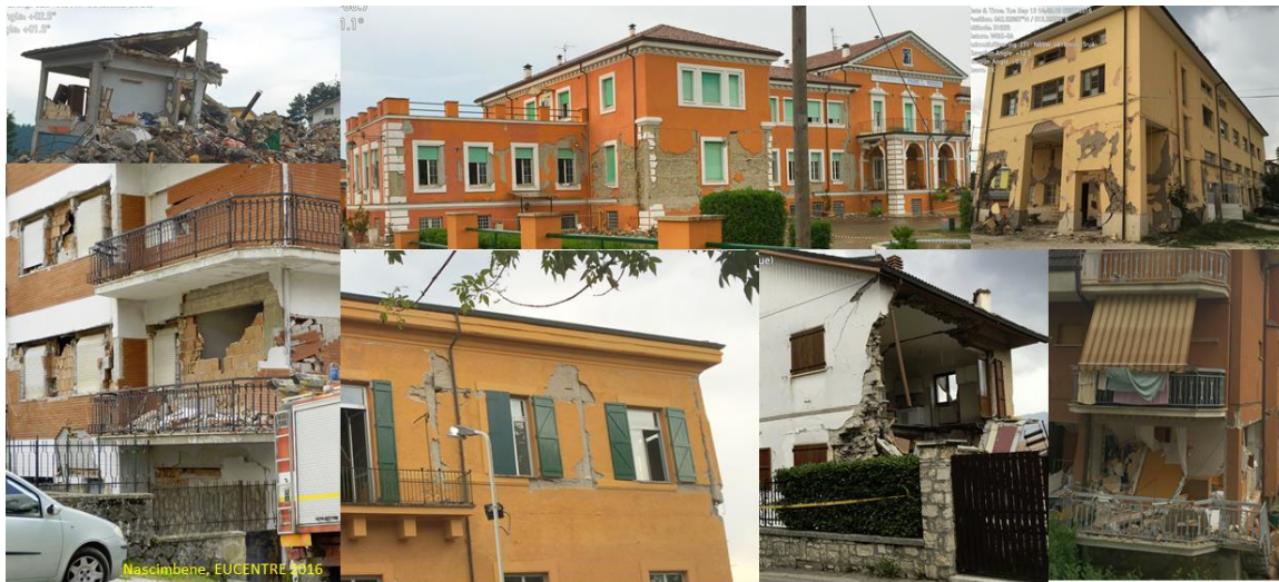
Figure 8. Representative Buildings and Damage in Periphery of Amatrice, September 2016
