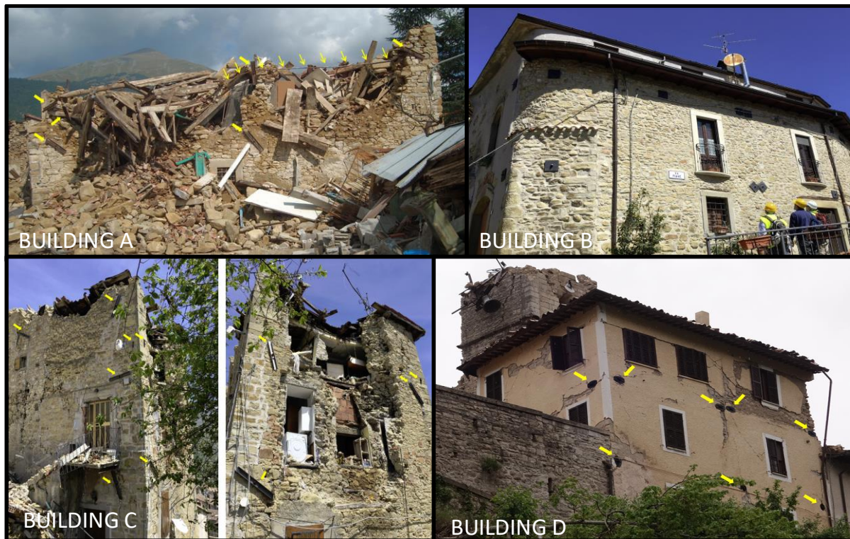
Figure 14. Strengthened Stone Masonry Buildings
