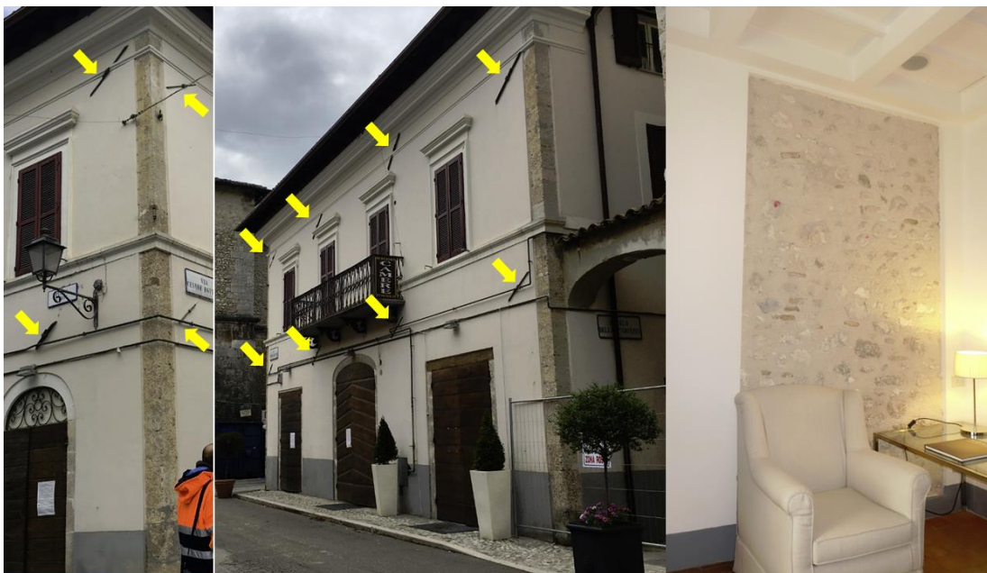
Figure 16. Example of Strengthening with Reinforced Plaster, Hotel Seneca in Norcia
