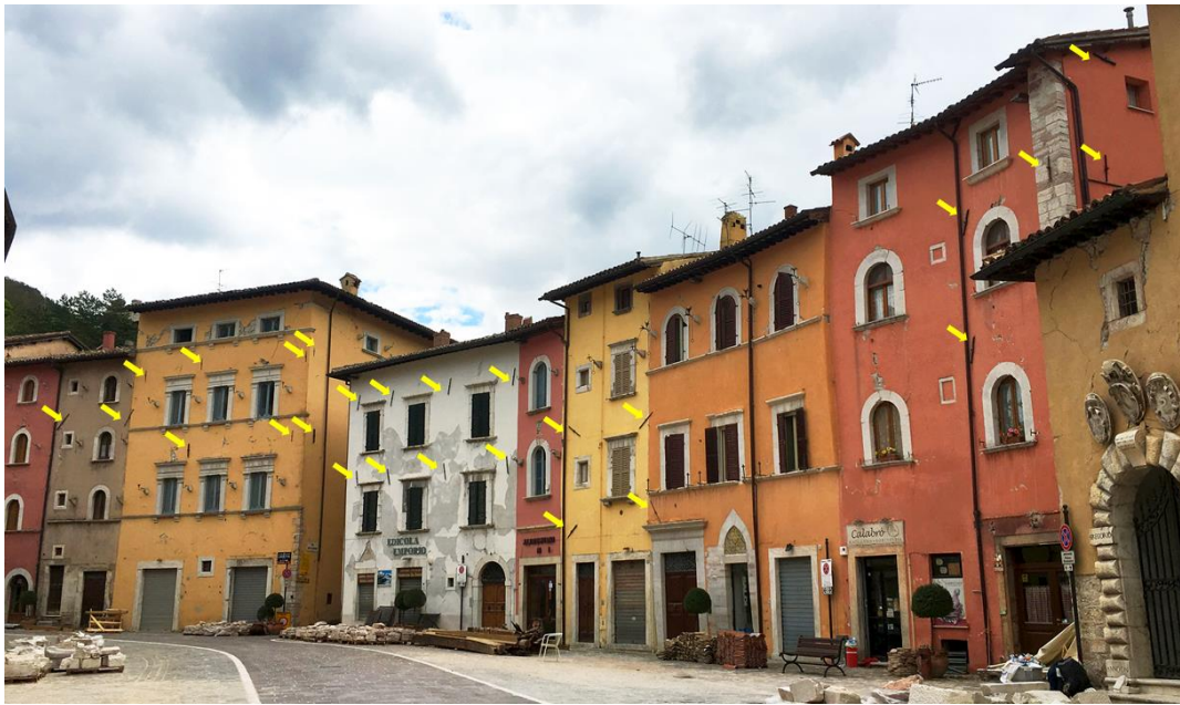
Figure 3. Wall Ties in the town of Visso in May 2017
