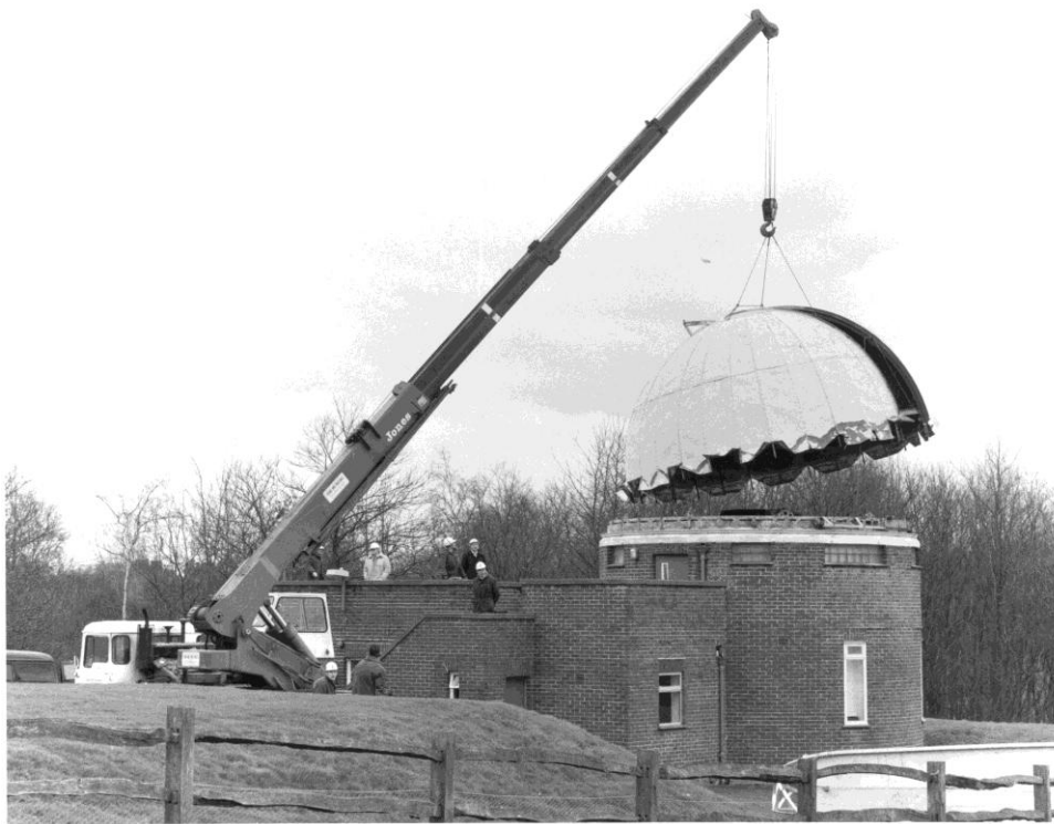
Figure 5.1 Removal of the solar dome in 1981 prior to installation of the clamshell dome.
