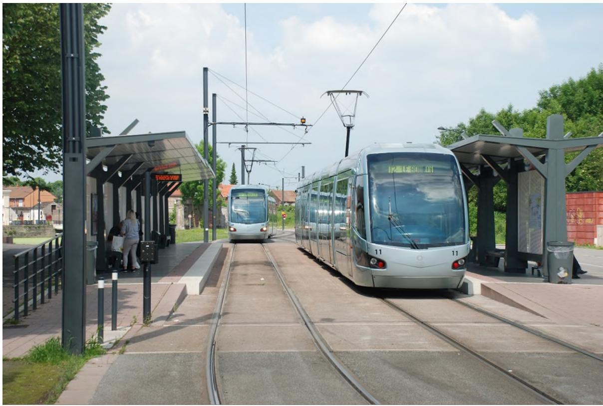
**Figure 2: Valenciennes, tram double-tracking at stations, and single track beyond**
