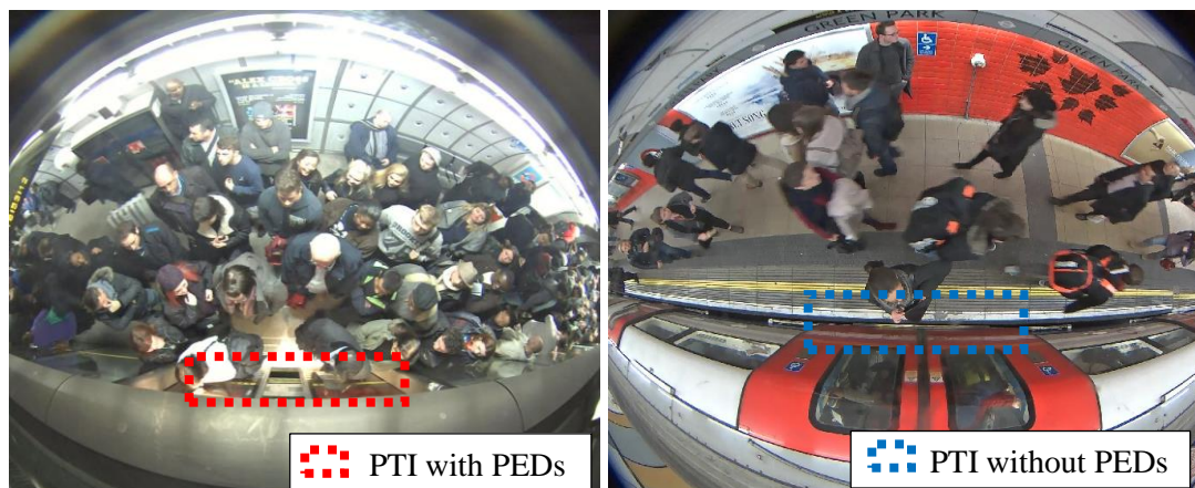
Figure 3-7: Platform train interface (PTI) with (left) and without (right) PEDs at LU stations.
