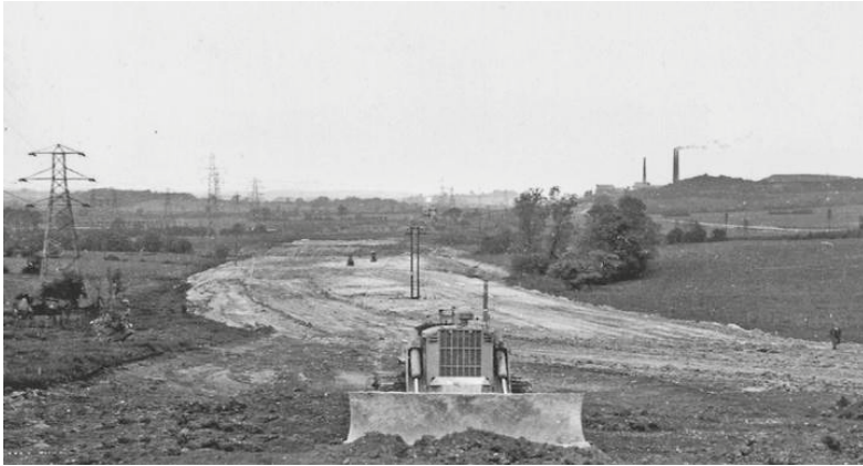
Figure 3.2 The construction of the M1 motorway through Bedfordshire in 1959 is marked by a swathe of bare earth, cleared and levelled by an army of machines such as the bulldozer prominent in the foreground. Source: photograph taken by Ben Brooksbank and reproduced by permission of the photographer.
