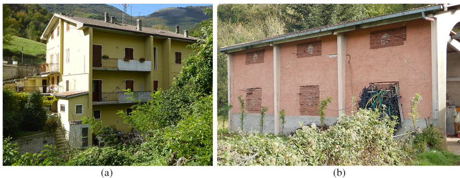
Fig. 16 a Building ID 41 in Arquata, Long. 42,46,33.64N Lat. 13,17,37.88E; b Building ID 5 in Grisciano (Accumoli municipality), Long. 42,43,51.57N Lat. 13,16,11.676E; Source EEFIT (2016)
