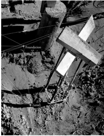
Foundation Construction in Sand – Open City, Chile.
