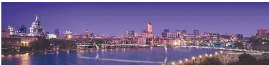
Figure 7: The Millennium Bridge wobbled alarmingly when it was opened, due to the large number of pedestrians crossing it.
