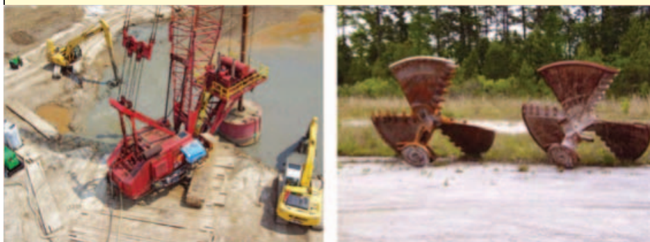
Figure 9. Soil mixing equipment (left) and mixing was completed using 3 m diameter augers (right) – Photos' credit: Professor Charles Shackelford (CSU).
