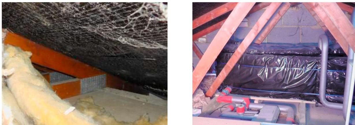
Figure 2: a) insulation missing above ceiling near eaves b) lack of insulation beneath cold water tank.
