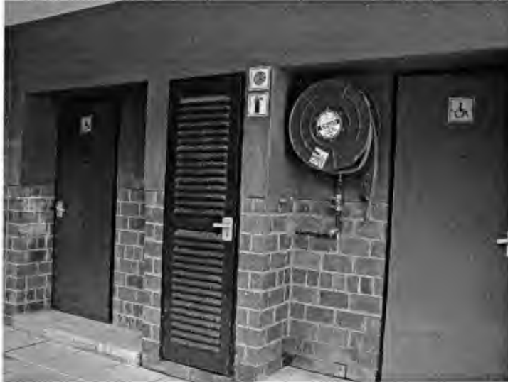
Image 24: 06K03a: Simunye Secondary: Toilets for people with physical disabilities
