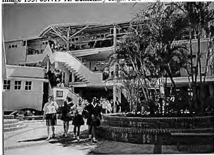
Image 133: 031419-X: Centenary High: AM Wing and refurbished courtyard with drinking fountain
