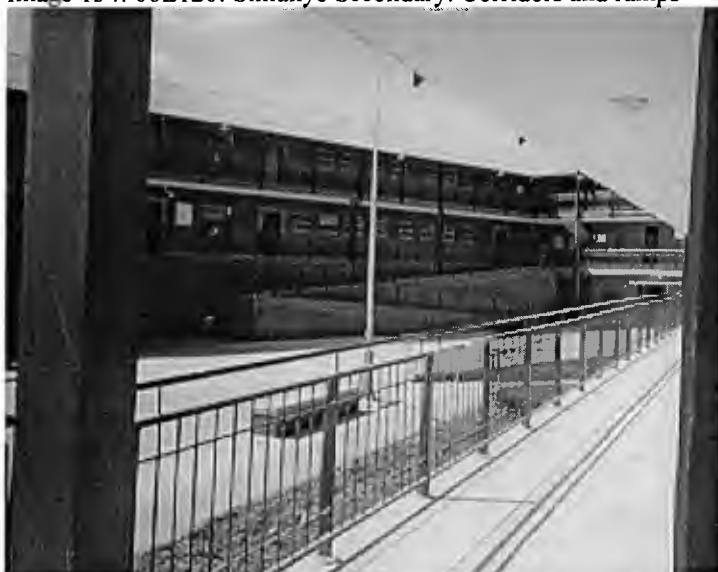
Image 134: 06L120: Simunye Secondary: Corridors and ramps
