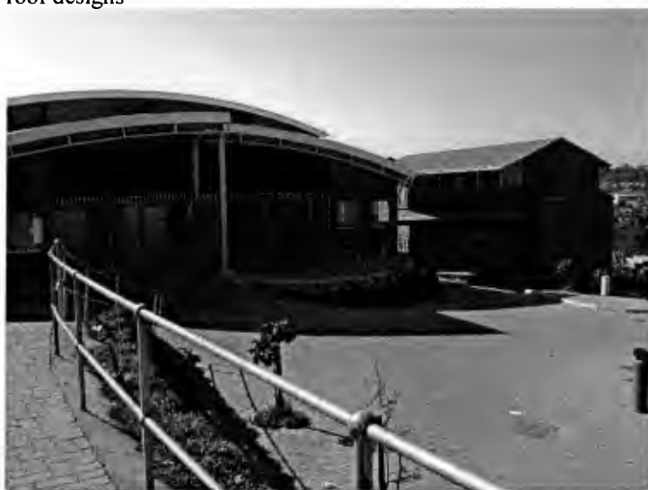
Image 138: 06K14c: Simunye Secondary: Different institutions and functions signalled in the contrasting roof designs
