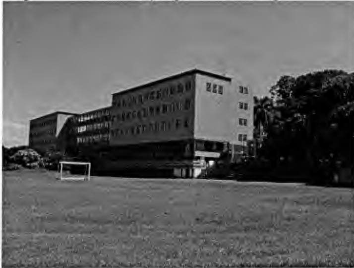
Image 8: 03K19d: Centenary High: Classroom wings and catwalks built in the 1970s
