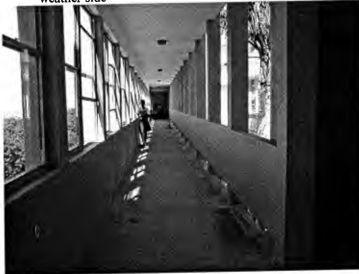
Image 13: 03K17e: Centenary High: 1970s high catwalks between classroom blocks, glazed on exposed weather side
