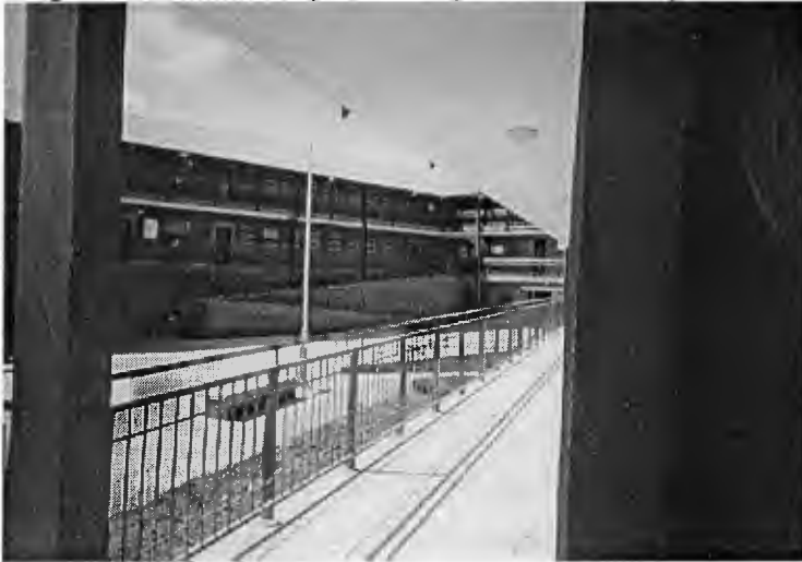
Image 25: 06L120: Simunye Secondary: Wheelchair ramps to access classrooms
