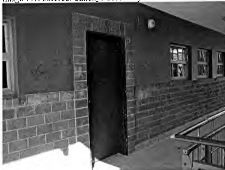
Image 141: 06K16b: Simunye Secondary: Brickwork at each classroom entrance
