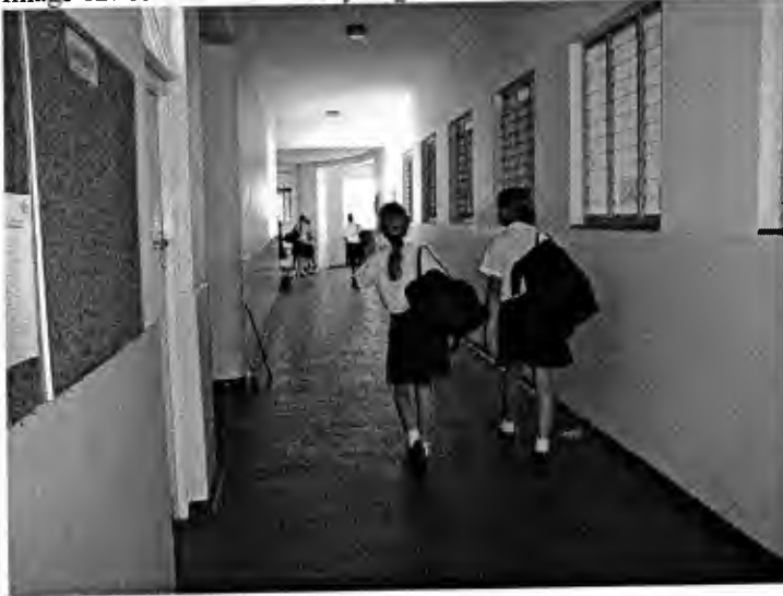
Image 12: 03K17b: Centenary High: 1930s enclosed corridor and modified classroom louvre windows
