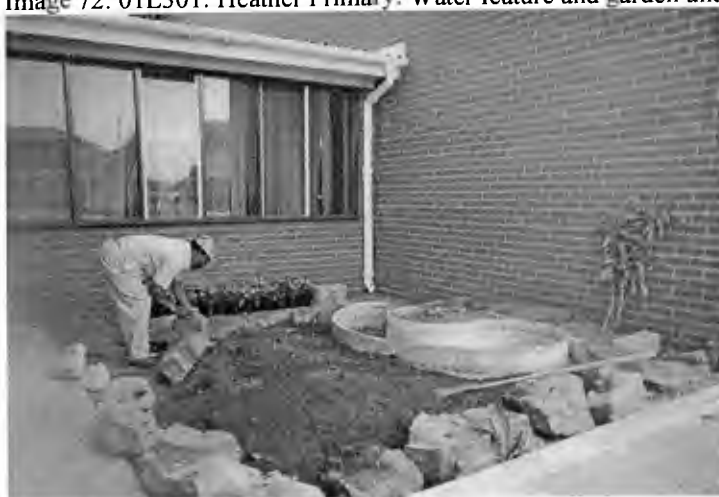
Image 72: 01L301: Heather Primary: Water feature and garden under construction
