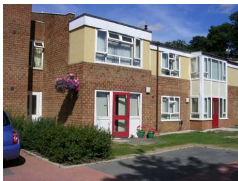
Figure 37: Patio door opening into the open court yard
