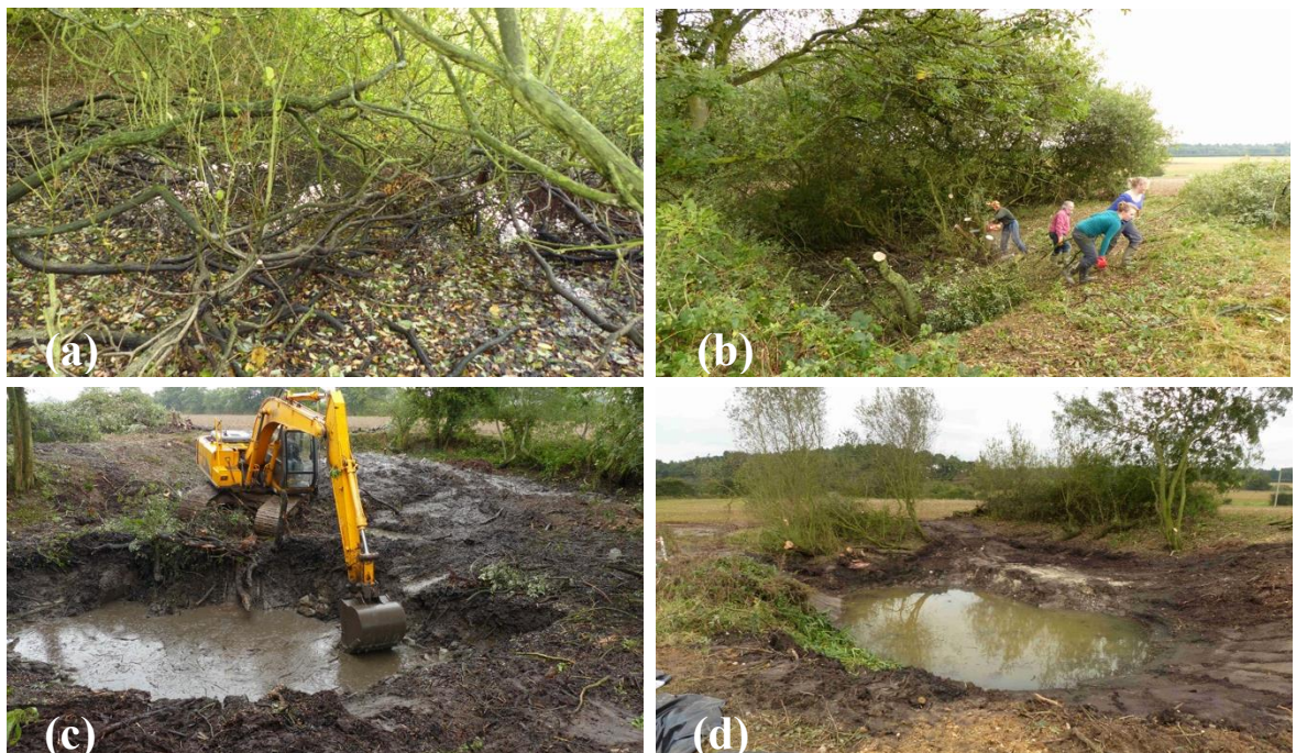
Figure 48 – Restoration of STRE in Oct. 2013. (a) Inside the pond, prior to restoration. (b) Beginning tree clearance. (c) Removing the surface layers of unstable, anoxic sediment, which had built-up during the overgrown pond phase. (d) Final profile of the restored pond. The lower layers of dark pond sediment were left in the basin to provide a source of propagules. The white marl clay, which forms the pond base, has been exposed in some areas, as can be seen towards the back of the pond.
