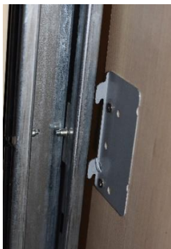
Figure 3. Connector devices used in the partitions
