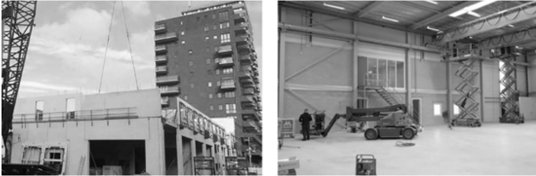
FIGURE 11 Under-construction housing tower building project of case B (left), and the interior of utility building of case C (right).
