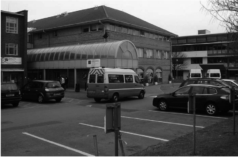
Figure 6.5: Sussex Downs College – unsatisfactory buildings surrounded by unattractive parking (photo courtesy of van Heyningen and Haward Architects)
