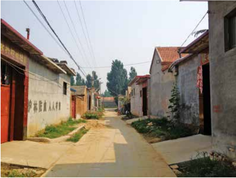
Fig. 1.3 Houses in the ‘old’ part of a village
