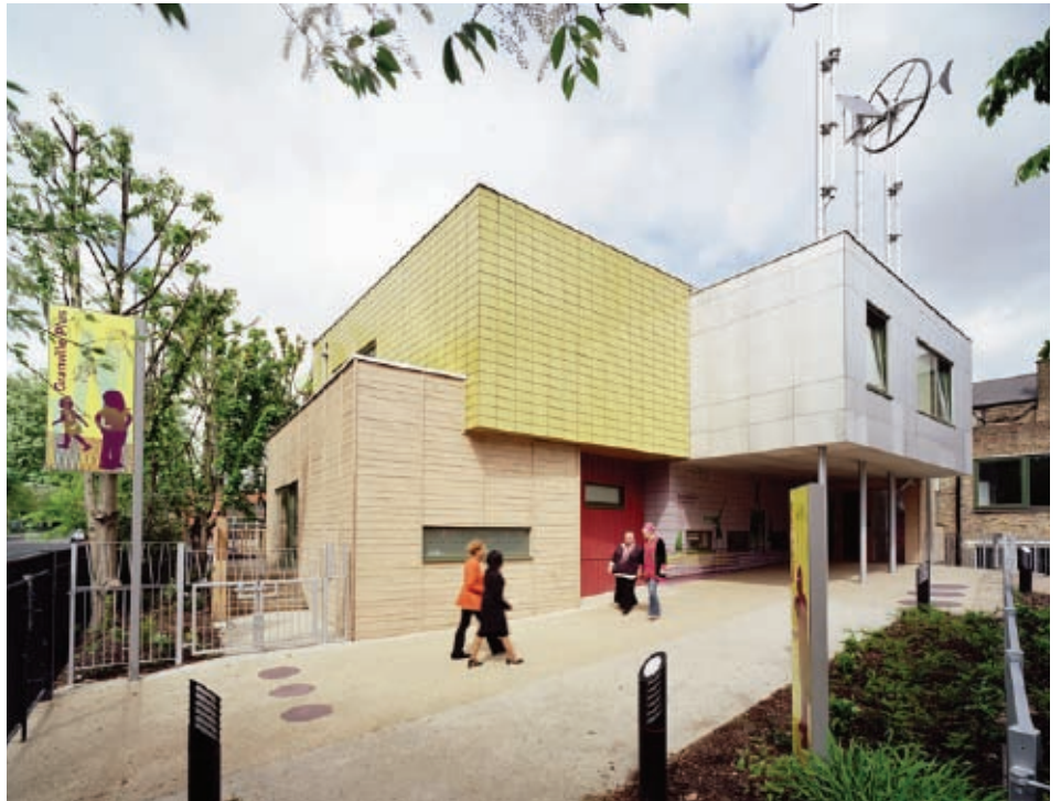
Clear, colourful, bold: a good children's centre will show you what it is from the street
