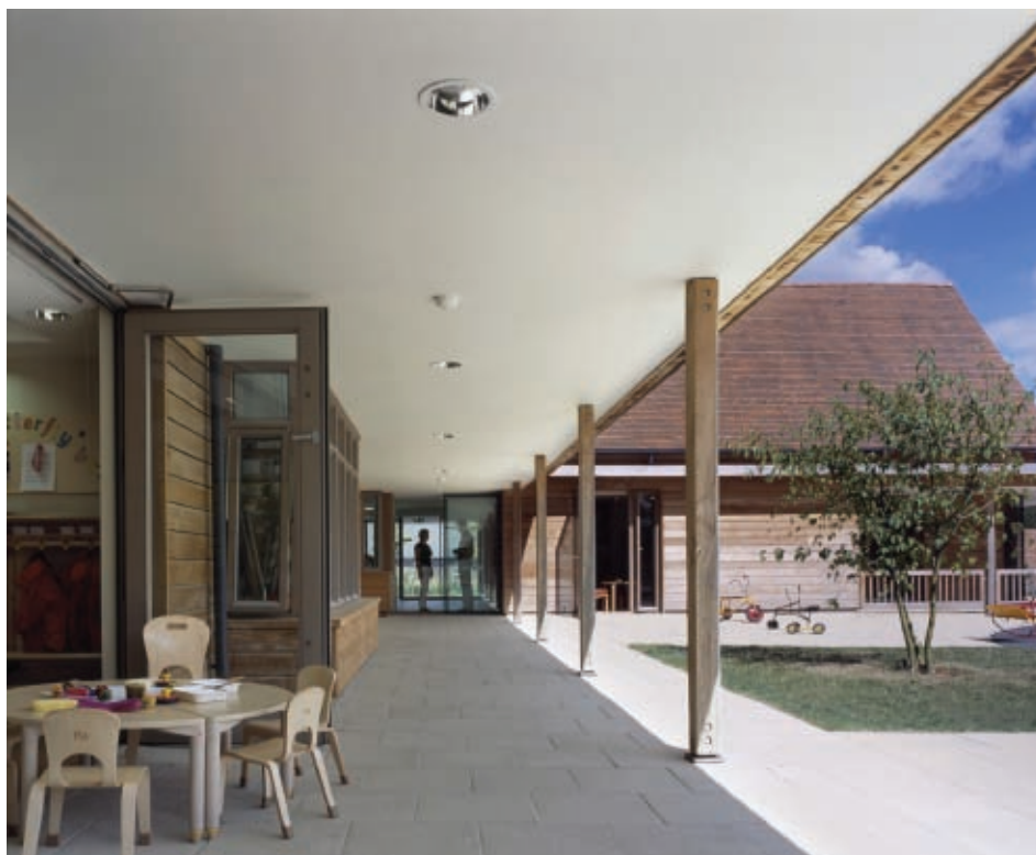
Level thresholds at entrances make the centre accessible and reduces the trip hazards for young children
