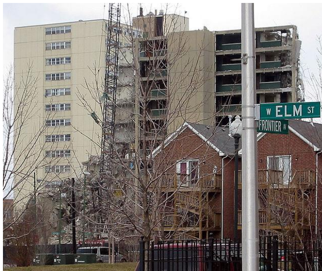
William Green Homes, under demolition. Payton Chung 2005
