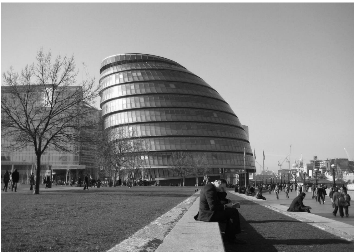
Figure 9. The GLA building in Potters Fields.
