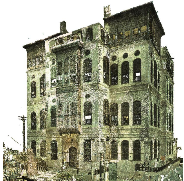
Figure 2: 3D LiDAR point cloud of Nasif Historical House.
