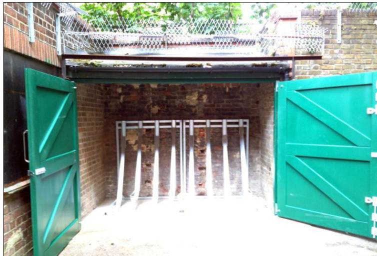
Figure 6.3 The 'small' cycle parking at Lissenden Gardens
