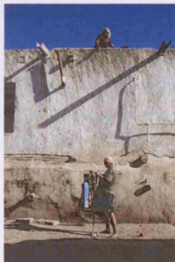
Fig. 56. Preparing to hoist buckets of prepared earth to the roof for maintenance application (UZ02_0106).
