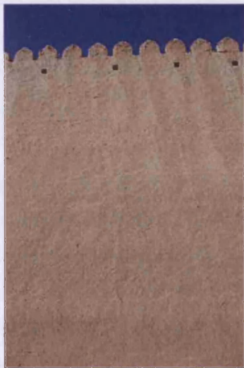
Fig. 87. Localised water run off at the base of reconstructed crenellations, Khiva, Uzbekistan (UZ01_0067).
