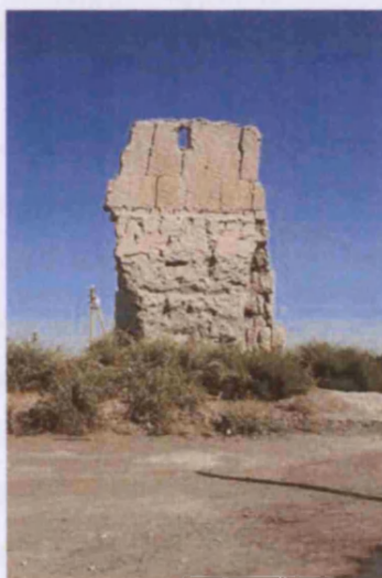
Fig. 74. Differential erosion between lifts and construction 'seams' on paksha wall Bukhara, Uzbekistan (UZ02_0007).
