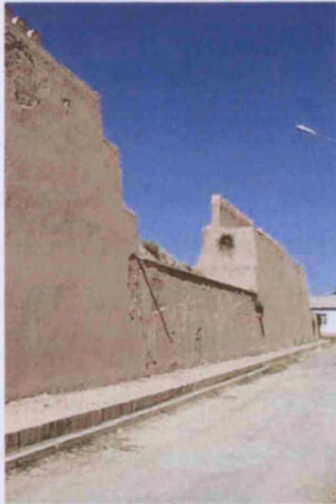
Fig. 144. Encapsulation using harder replacement materials, Shahrissabz city walls (UZ03_0028).
