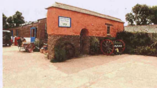
Fig. 20. Cob frontage, Gear Farm Shop, Cornwall United Kingdom.
