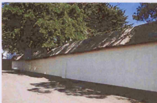
Fig. 21. Cob wall, East Budleigh, Devon, United Kingdom.
