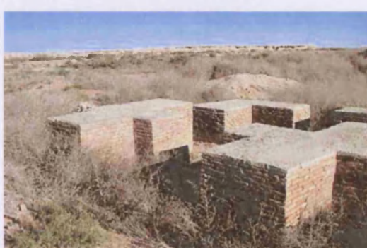
Fig. 129. Encapsulation with harder, replacement materials, Merv (TM01_0112).
