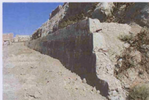
Fig. 136. Encapsulation within paksha wall, Bukhara city walls (UZ02_0017).
