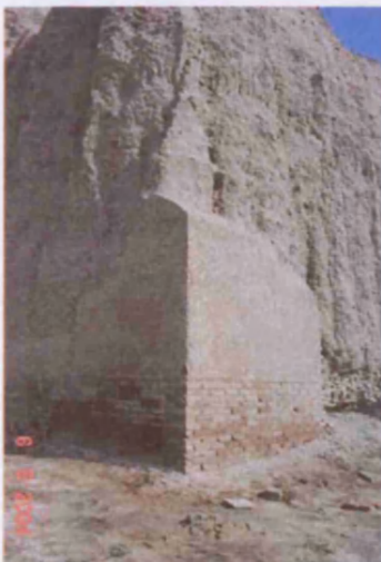
Fig. 172. Fired brick and mudbrick undercut repair, Merv (TM01_0076).
