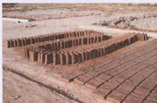
Fig. 9. General view of mudbricks stacked on their end to dry, Yazd, Iran (IR07_0069)
