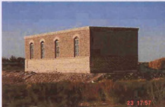
Fig. 58. House under construction on a raised earth platform utilising fired brick and mudbrick (TM01_0061)
