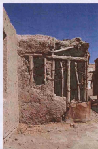
Fig. 37. Abandoned sintch building, with earth infill, Khiva, Uzbekistan (UZ01_0047).
