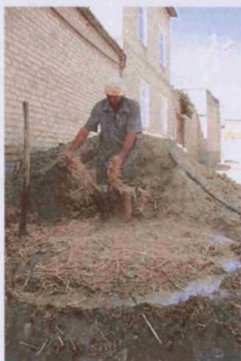
Fig. 52. Preparing the earth mix for maintenance by adding wheat straw, Bukhara, Uzbekistan (UZ02_0100).
