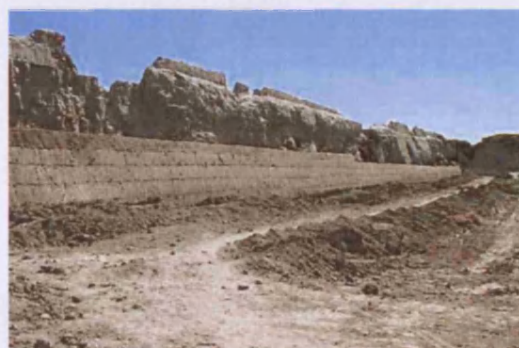
Fig. 137. Encapsulation within paksha wall, Bukhara city walls (UZ02_0056).
