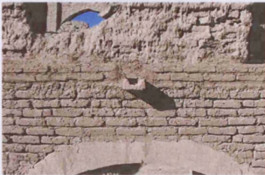
Fig. 48. Reconstructed drainage spout, Bam, Iran (IR10_0013).
