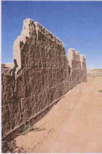
Fig. 29. Modern tall and thin paksha wall for unfinished industrial buildings, Merv, Turkmenistan (TM01_0120).
