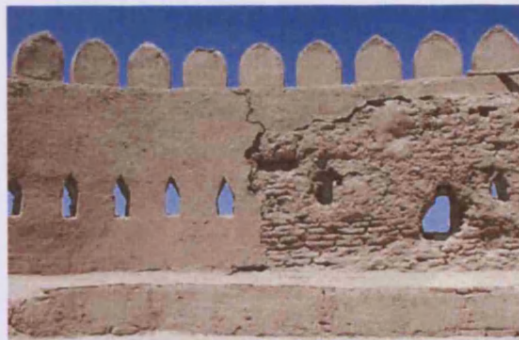
Fig. 134. Encapsulation using cement render, Khiva (UZ01_0017).
