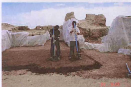
Fig. 109. Compacting bulk fill in lifts for long-term backfilling at Merv (TM01_0030).
