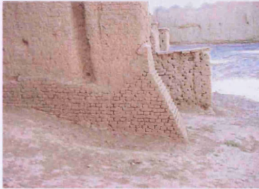
Fig. 170. Mudbrick undercut repair, Merv (TM01_0001).
