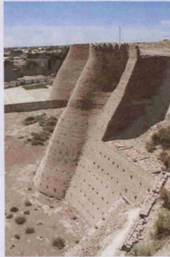
Fig. 141. Encapsulation using harder replacement materials, Bukhara Ark (UZ02_0076).
