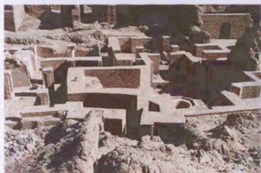
Fig. 123. Encapsulated excavated walls, Bam (IR10_0044).
