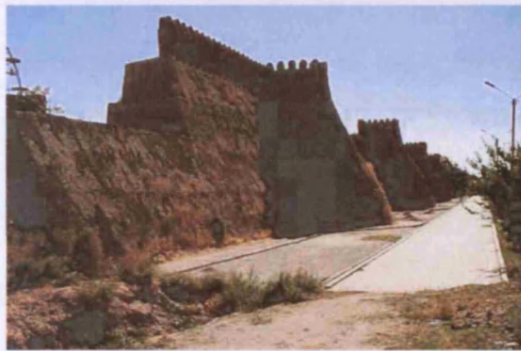
Fig. 145. Encapsulation using harder replacement materials, Shahrissabz city walls (UZ03_0035).
