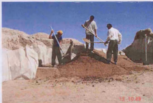
Fig. 111. Preparing drainage slopes for long-term backfilling at Merv (TM01_0025).
