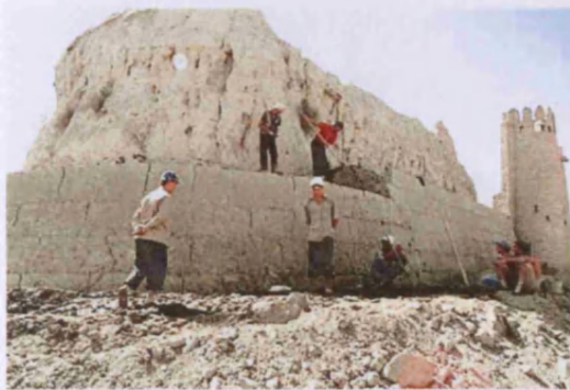
Fig. 139. Encapsulation within paksha wall, Bukhara city walls (UZ02_0137).
