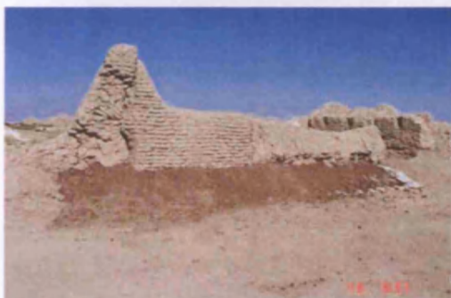
Fig. 165. Drainage slope incorporated into backfilling, Merv (TM01_0029).
