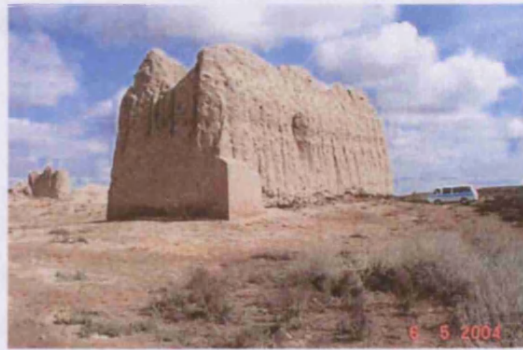
Fig. 173. Fired brick and mudbrick undercut repair, Merv (TM01_0075).
