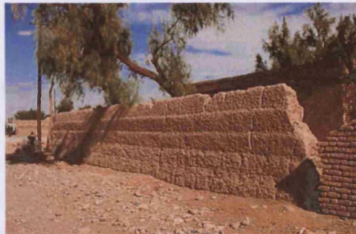
Fig. 84. Chineh wall with eroded wall top and drip gullies associated with increased humidity from adjacent vegetation, Shahdad, Iran (IR34_0013).
