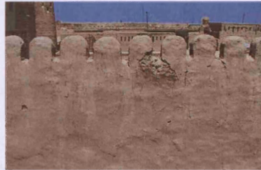
Fig. 88. Localised water run off at the base of reconstructed crenellations, Khiva, Uzbekistan (UZ01_0028).
