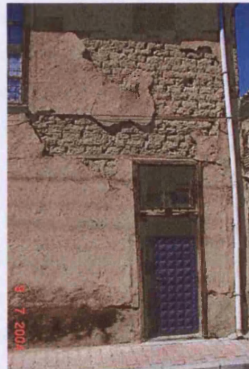
Fig. 42. Fallen cement and earth plaster revealing damage to mudbrick wall core, Konya, Turkey (TK06_0032)
