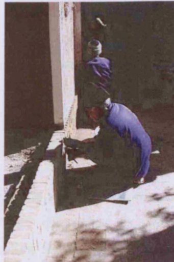
Fig. 189. Restoration using new replacement, and earthen materials, Bam (IR10_0021).
