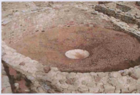
Fig. 168. Surface water collection for backfilled rooms, Aztec (US01_0017).
