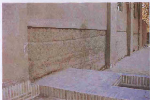
Fig. 122. Encapsulated chineh wall, Yazd (IR07_0083).
