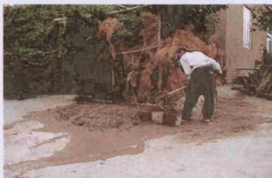
Fig. 51. Preparing the earth mix for maintenance of the exterior surface, Khiva, Uzbekistan (UZ01_0087).
