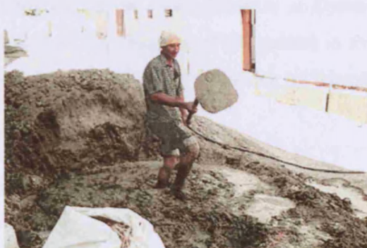
Fig. 55. Mixing the earth, water and wheat straw mix for maintenance, Bukhara, Uzbekistan (UZ02_0151).
