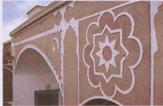
Fig. 41. Restored earth and decorative gaunch plaster, Yazd, Iran (IR07_0034).
