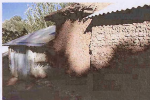
Fig. 38. Variety of earth walls, including sintch with hand formed earth balls as infill, Zerafshan Mountains, Uzbekistan (UZ03_0070).
