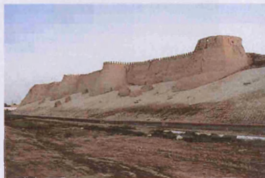
Fig. 135. Encapsulation using harder replacement materials, Ichin Kala wall, Khiva (UZ01_0073).
