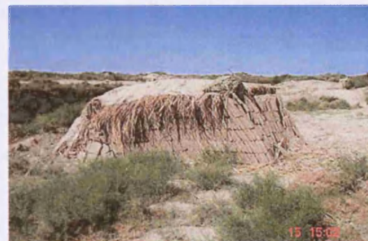
Fig. 14. Stack of dried mudbricks with reed and mud plaster thatch to protect from rain, Merv, Turkmenistan (TM01_0063).
