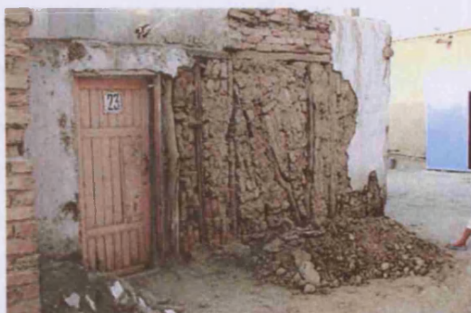
Fig. 54. Render removed from sintch wall render for maintenance, Bukhara, Uzbekistan (UZ02_0109).
