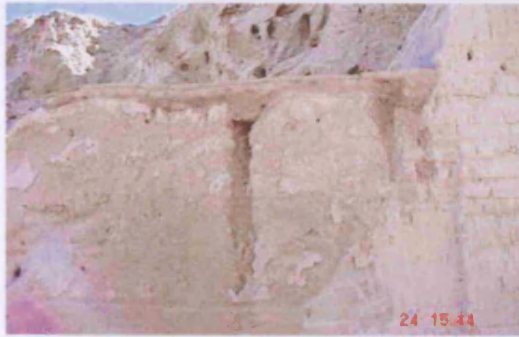
Fig. 162. Earth mortar plugging drainage gullies, Merv (TM01_0131).
