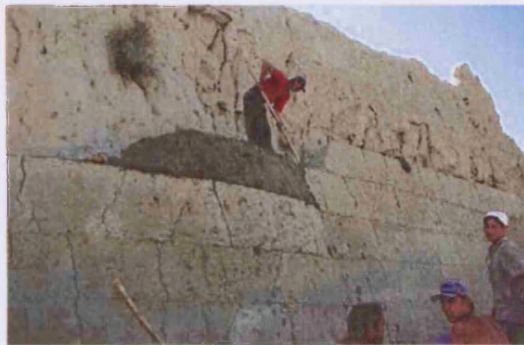
Fig. 26. Construction of paksha wall for conservation work, Bukhara, Uzbekistan (UZ02_0034). Each earth 'lift' is pared down with a spade.
