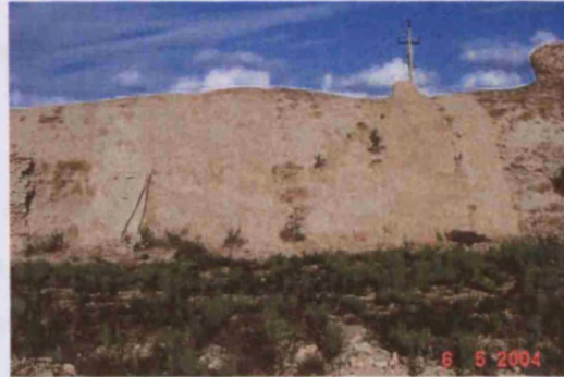
Fig. 147. Condition of experimental encapsulation work using geotextile, and earthen plasters after 1 year, Merv (TM01_0079).
