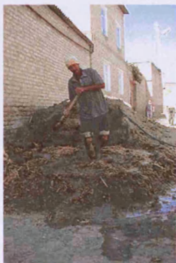
Fig. 53. Mixing the earth, water and wheat straw mix for maintenance, Bukhara, Uzbekistan (UZ02_0101).
