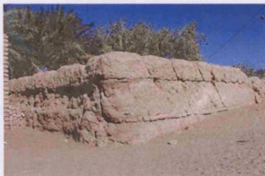
Fig. 75. Differential erosion of chineh lifts, Shahdad, Iran (IR34_0022).
