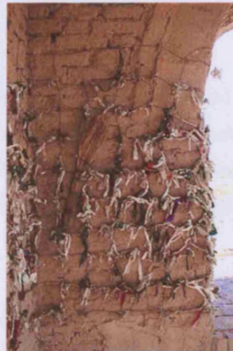
Fig. 148. Prayer rags tied onto wire exposed after collapse of cement render used in encapsulation/restoration work, Kyz Bibi Mausoleum, Merv (TM01_0105).
