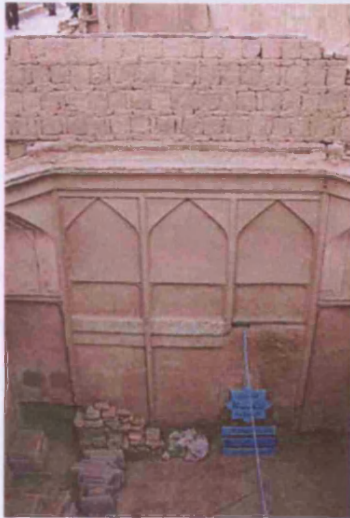
Fig. 187. Structure being restored, using mudbricks, Yazd (IR07_0056).
