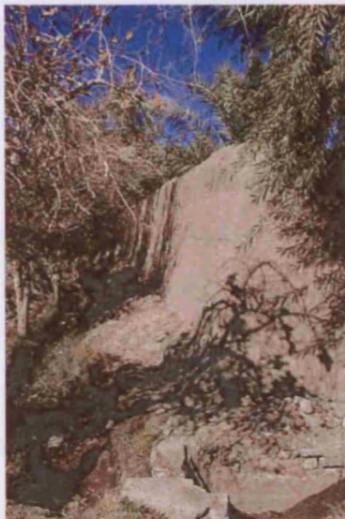
Fig. 83. Chineh wall with eroded wall top associated with increased humidity from adjacent vegetation, Bam, Iran (IR10_0054).
