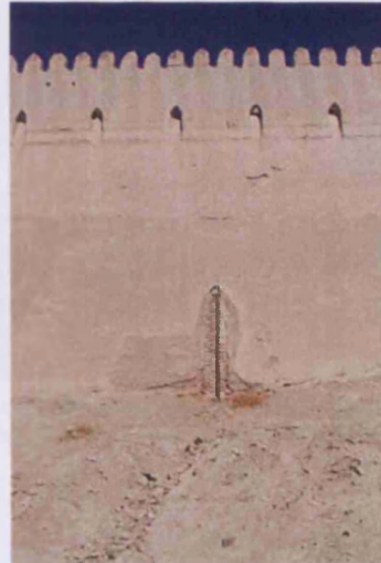
Fig. 49. Repaired vertical drain, and area of water damage, Bam, Iran (IR10_0024).
