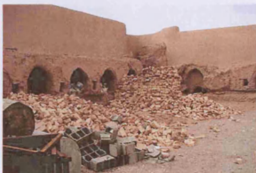
Fig. 127. Encapsulation with replacement materials, and coated in earthen plaster, Shemsh (IR36_0008).
