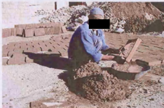
Fig. 8. General view of mudbricks being made for conservation work, Bam, Iran (IR10_0010)
