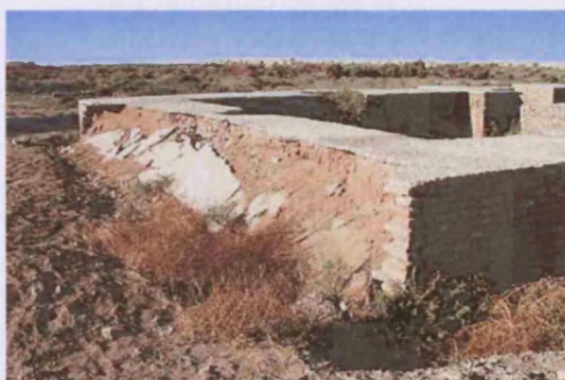
Fig. 128. Failure of harder, replacement encapsulation materials (and significant damage to surviving wall), Merv (TM01_0109).
