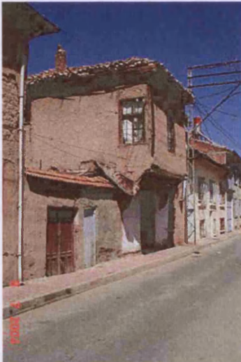
Fig. 40. Earth and cement based renders, Konya, Turkey (TK06_0033).
