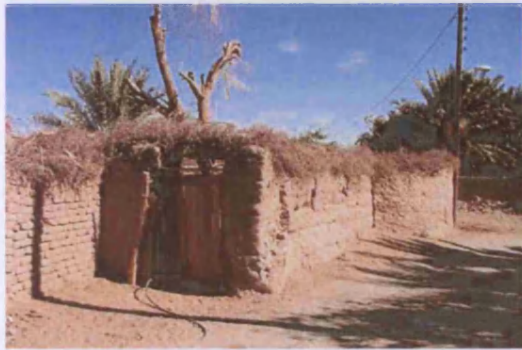
Fig. 116. Brush wood capping on top of chineh boundary wall, Shahdad (IR34_0027).
