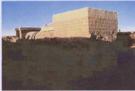
Fig. 119. Fired brick, cement, and tile capping experiments, Gonur (TM15_0052).
