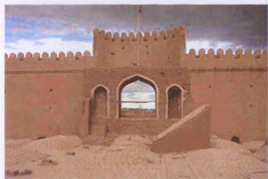
Fig. 125. Encapsulated and reconstructed walls, Rayen (IR35_0010).
