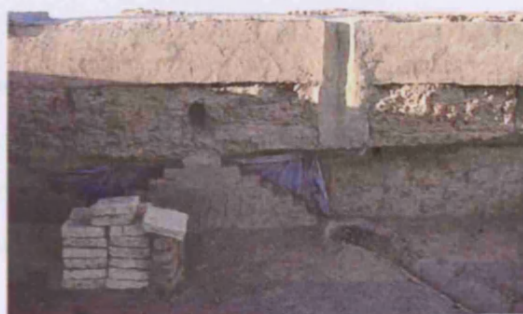
Fig. 175. Experimental undercut repair, Gonur (TM15_0051).
