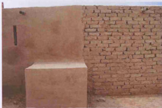
Fig. 130. Encapsulation and in situ reconstruction, using replacement and earthen materials, Nisa (TM02_0074).
