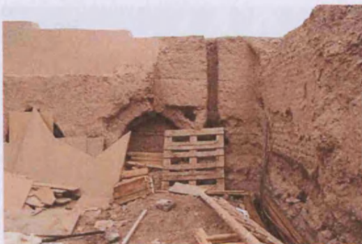
Fig. 126. Encapsulation with replacement materials, and coated in earthen plaster, Shemsh (IR36_0004).
