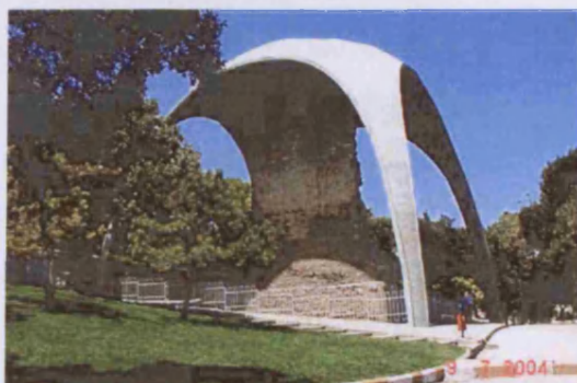
Fig. 201. Permanent concrete shell structure over Seljuk Palace, Konya (TK06_0001).
