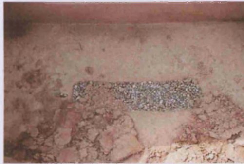
Fig. 166. Surface drain filled with aggregate, Nisa (TM02_0064).
