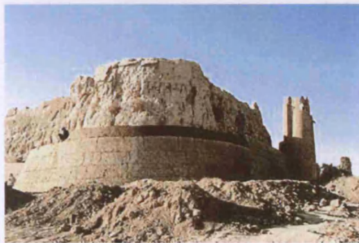
Fig. 140. Encapsulation within paksha wall, Bukhara city walls (UZ02_0145).
