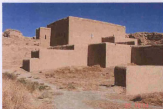
Fig. 131. Encapsulation and in situ reconstruction, using replacement and earthen materials, Nisa (TM02_0020).
