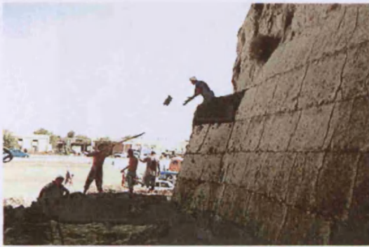
Fig. 23. Construction of paksha wall for conservation work, Bukhara, Uzbekistan (UZ02_0135). The prepared earth is thrown to the builder on the wall top.
