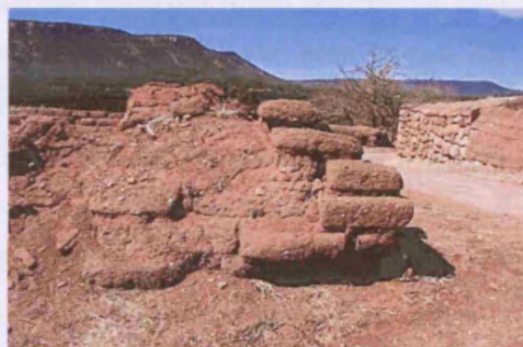
Fig. 154. Amended mudbricks used for encapsulation of wall, Pecos (US21_0010).
