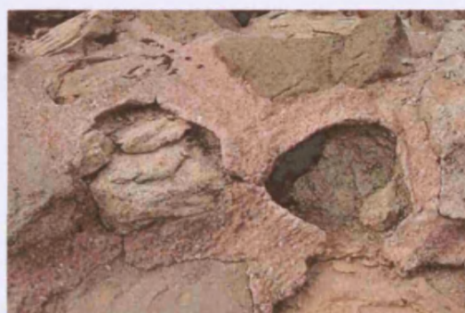
Fig. 155. Damage to stonework as a result of use of cement-amended mortar, Aztec (US01_0008).
