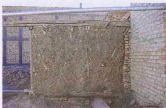
Fig. 35. Newly constructed sintch partition wall, with fired brick coated in earth render, Bukhara, Uzbekistan (UZ02_0093).
