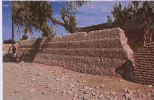
Fig. 27. Chineh boundary wall, Shahdad, Iran (IR35_0012).
