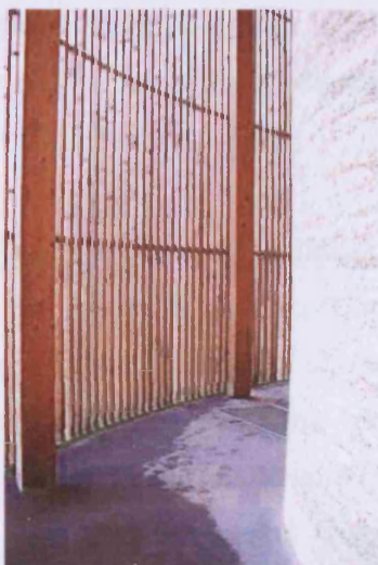
Fig. 16. Modern rammed earth wall at the Chapel of Reconciliation, Berlin (GM01_0011).
