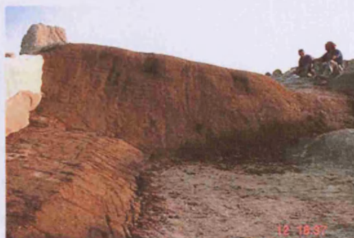
Fig. 112. Preparing drainage slopes for long-term backfilling at Merv (TM01_0072).
