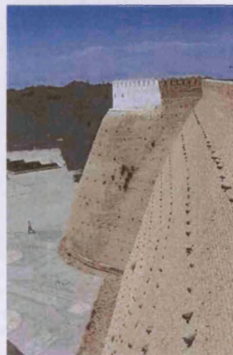
Fig. 142. Encapsulation using harder replacement materials, Bukhara Ark (UZ02_0081).
