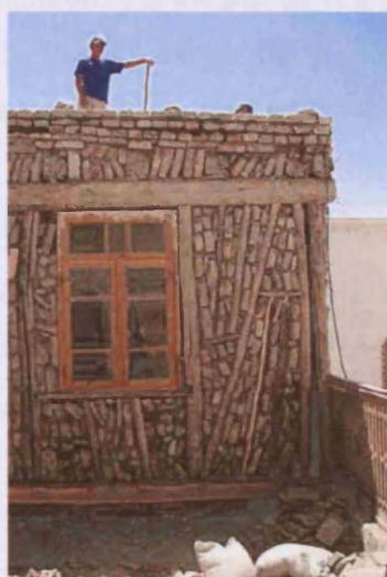
Fig. 34. Sintch building with fired brick infill between splayed timbers, Bukhara, Uzbekistan (UZ02_0069).
