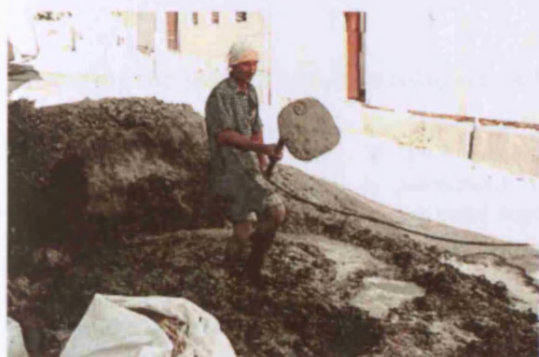
Fig. 177. Preparing earthen material for roof maintenance, Bukhara (UZ02_0151).
