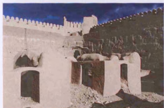
Fig. 124. Encapsulated excavated walls, Rayen (IR35_0004).
