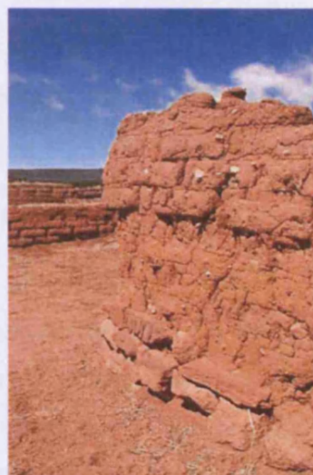
Fig. 153. Amended mudbricks for encapsulation of wall, Pecos (US21_0013).
