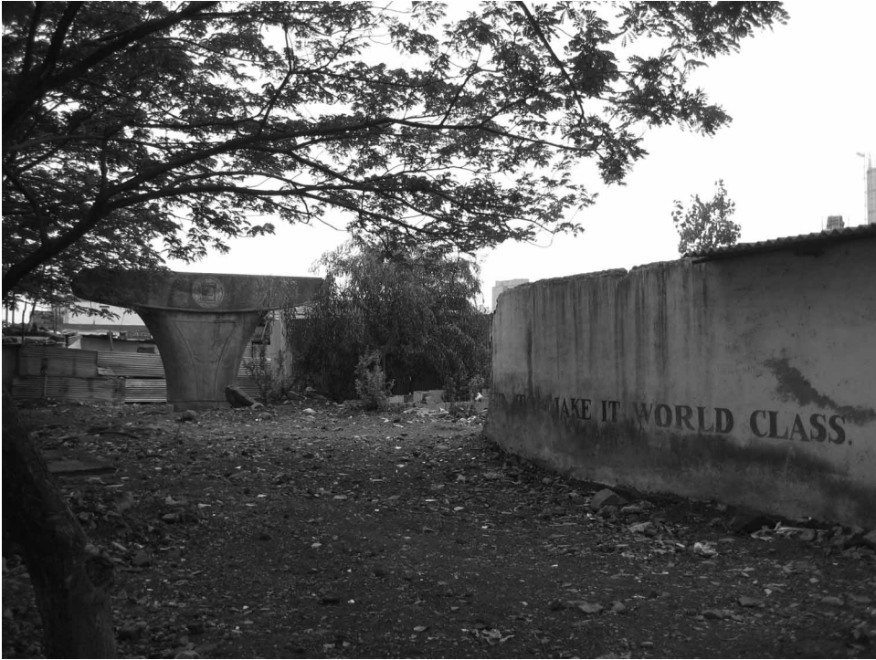
Figure 7 Flyover pier test site, Bandra–Kurla Complex, June 2009. Photograph by the author.
