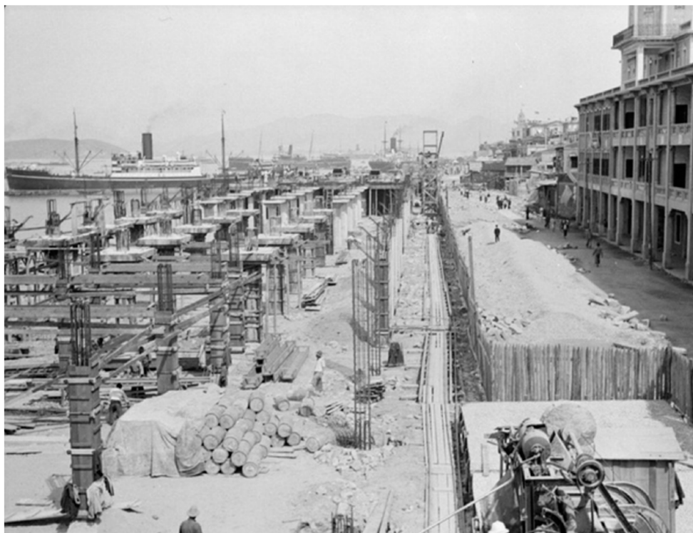
Figure 6. Construction of the Xiamen Bund (Source: collection by Swire, G. Warren, 1933–4; image courtesy of Special Collection [reference number: Sw08-088], University of Bristol Library [www.hpcbristol.net])
