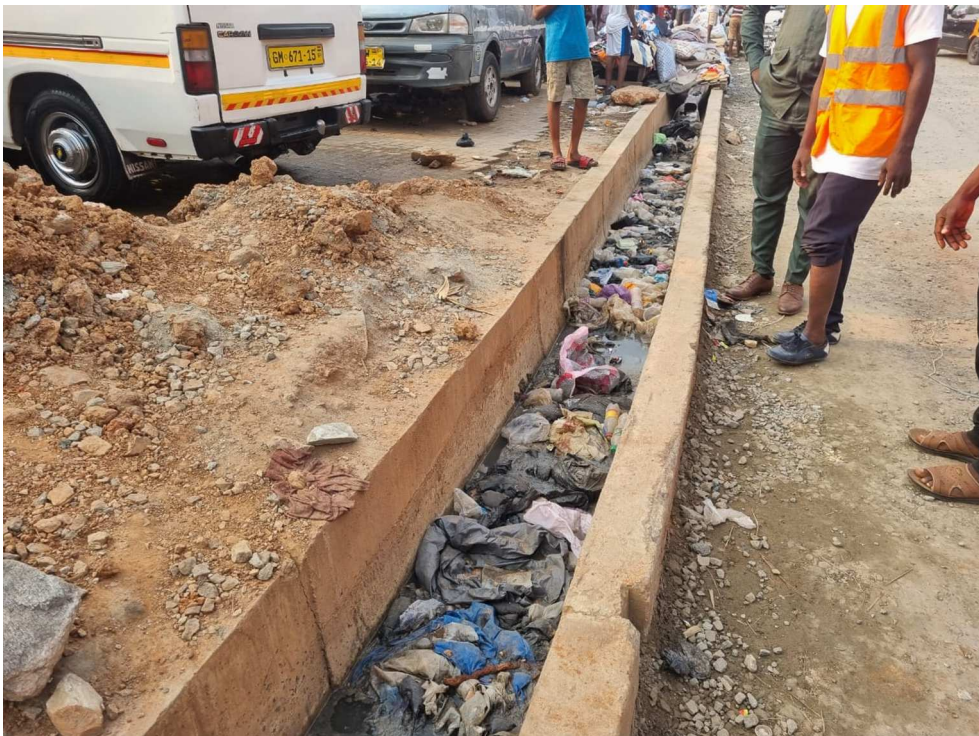
Figure 2. Choked drainage system in one of the GARID case study communities. Source: Fieldwork (2024).
