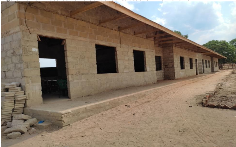
Figure 4-5 New Classrooms were under constructions in 2021 and 2022
