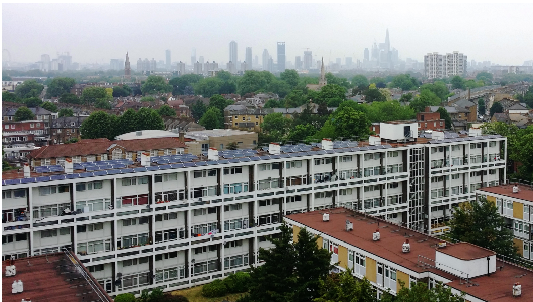
Figure 5.1: Elmore House Brixton (EDF, 2019).
