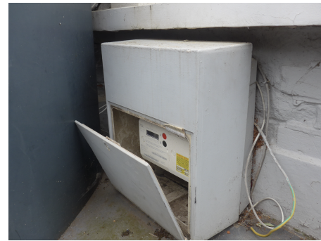
Figure 3: Barry's original energy meter, placed very low down to the ground.
