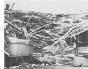
FIGURE 2. Plant area close behind and to the left of the CO 2 tank after failure.
