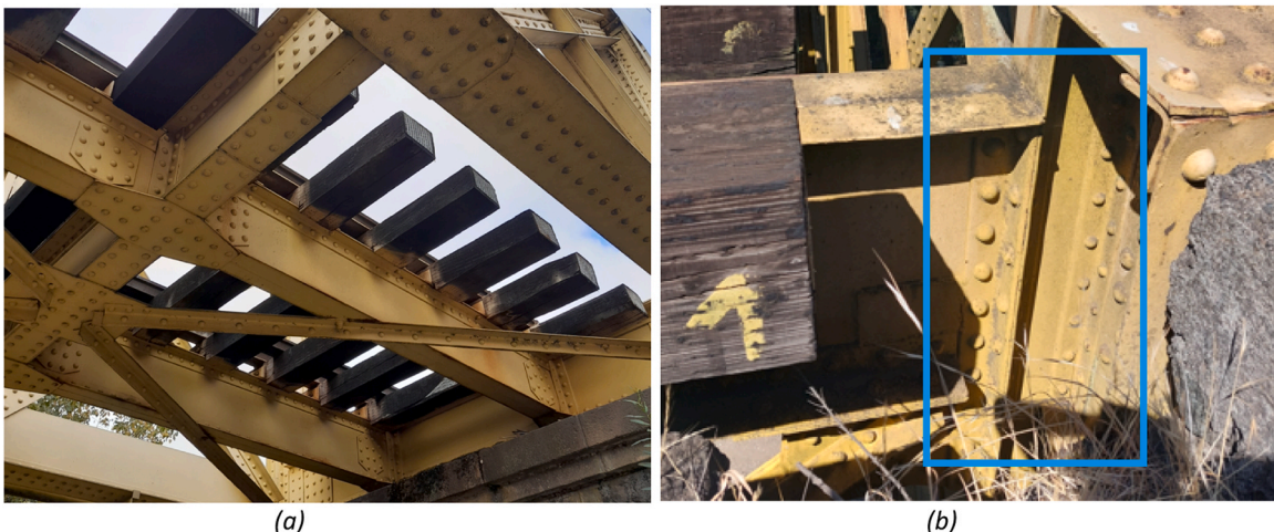
Fig. 1. Typical riveted double-angle connections in Chilean railway bridges. (a): Stringer-to-floor-beam connections; (b): Floor-beam-to-truss-girder connection.
