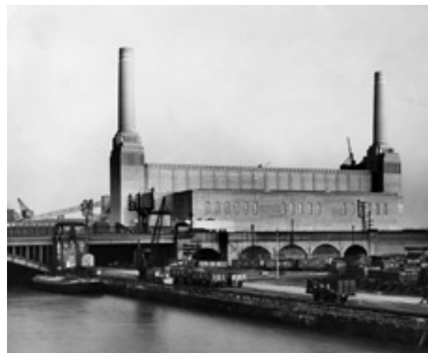
427. Battersea Power Station, west flank in 1933, with Battersea Wharf in the foreground
