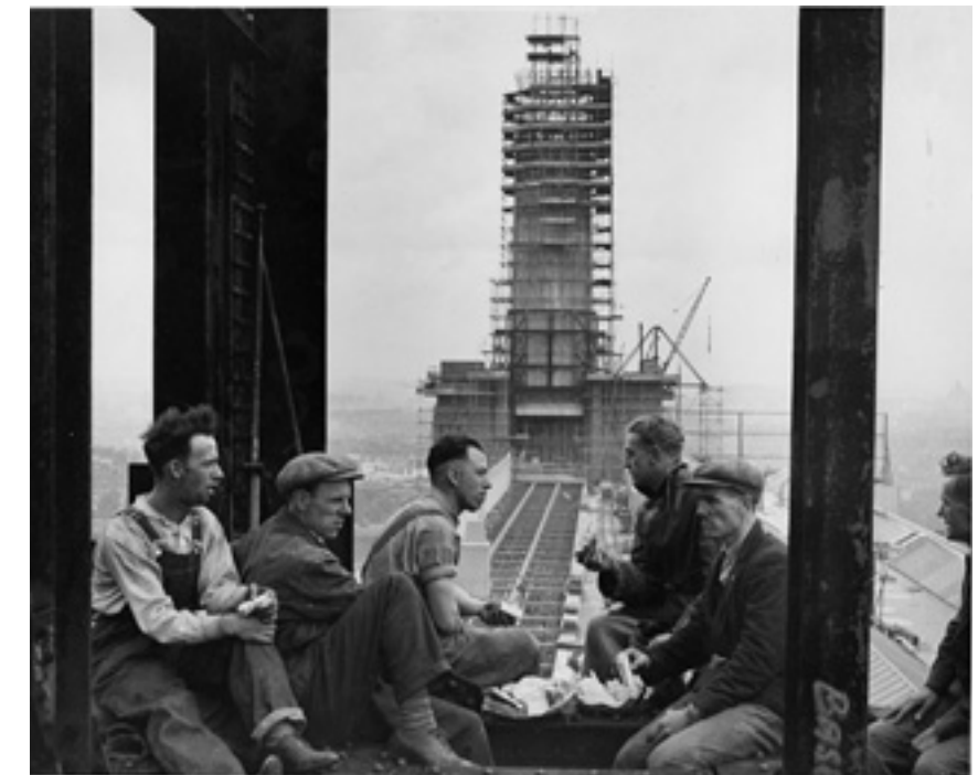
425. Battersea Power Station, lunch break on the roof of Station 'A' in 1931
