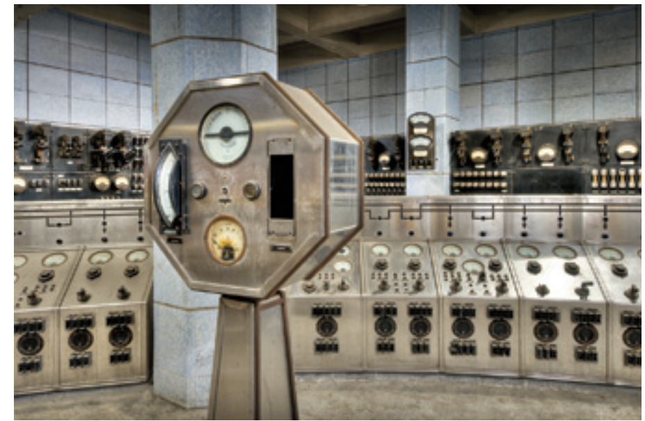
432. Battersea Power Station, Station 'B' Auxiliary Control Room in 2011
