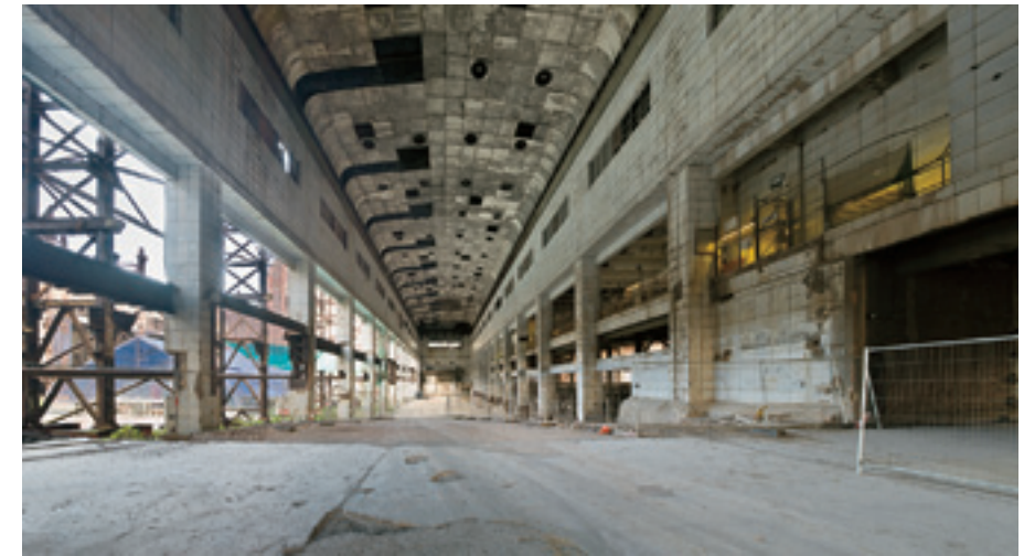
431. Battersea Power Station, Station 'B' Turbine Hall in 2011
