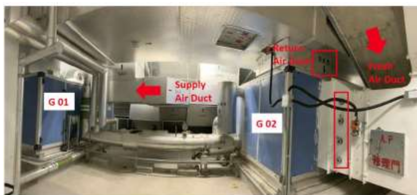
Figure A1. HVAC system arrangement in IAS lecture theatre
